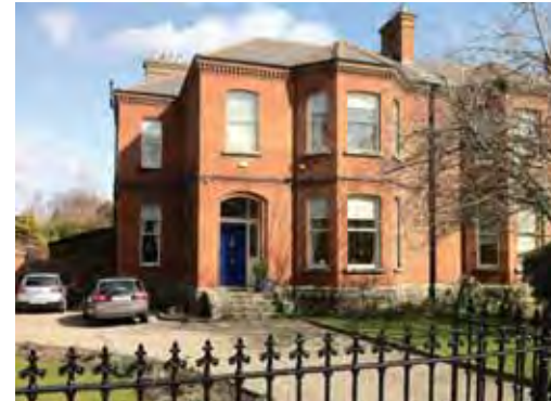
Houses along Park Avenue demonstrate the quality and variety of architecture prevalent throughout the Village.
