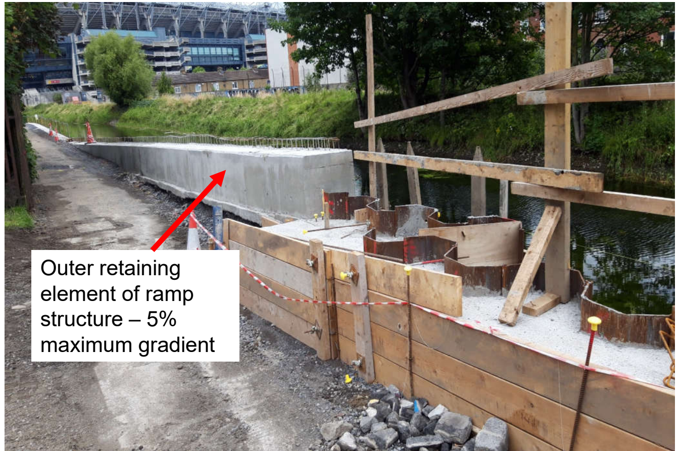
Clarke's Bridge west side ramp structure under construction
