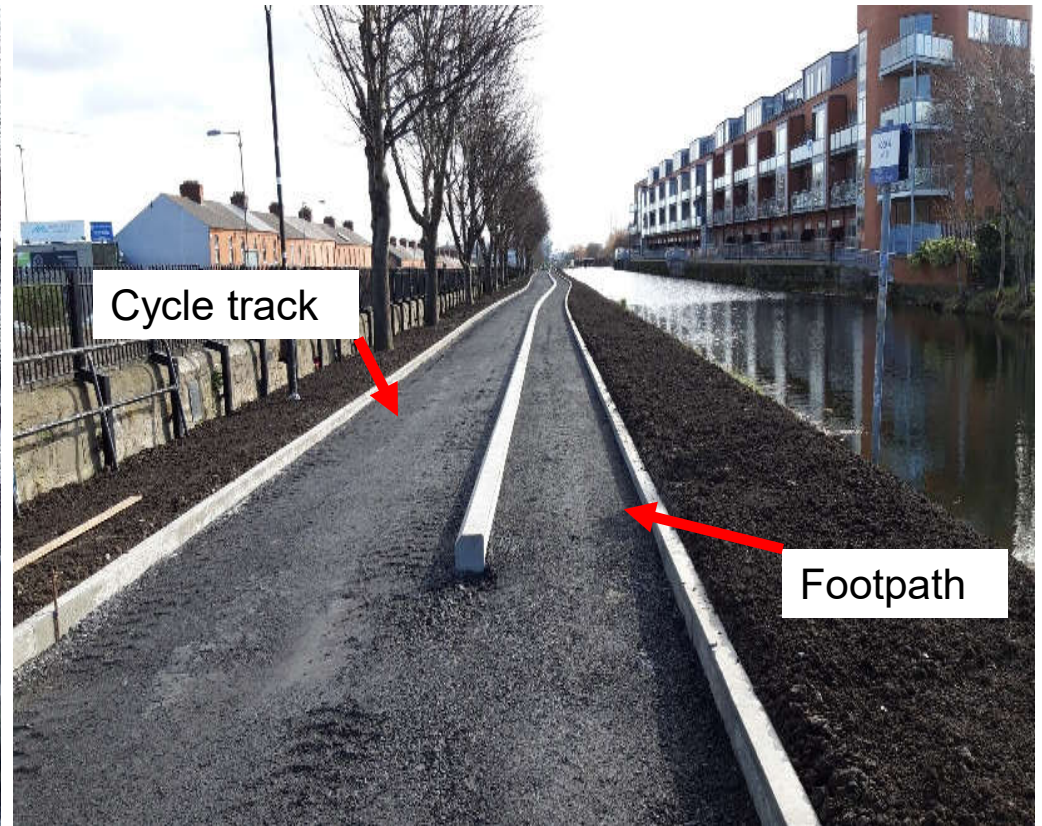
New kerbing works along south & north side towpath – the new kerb delineates the new cycle track and footpath
