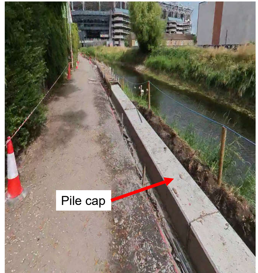
Sheet pile capping beam under construction to widen the footpath / cycle track area
