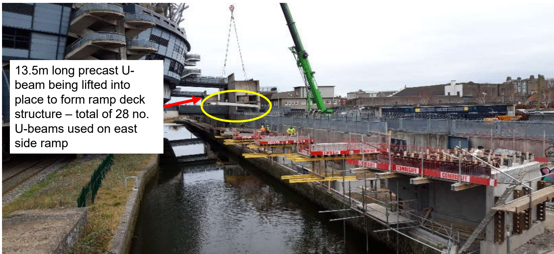
Russell St. east side ramp deck beams being lifted into place using a 250 tonne mobile crane
