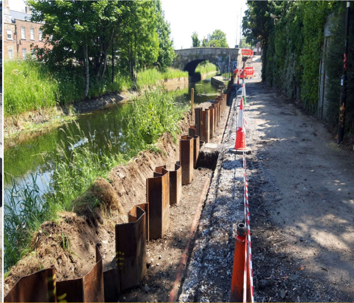
New sheet piles installed between Bloody Sunday Bridge & Clarke's Bridge
