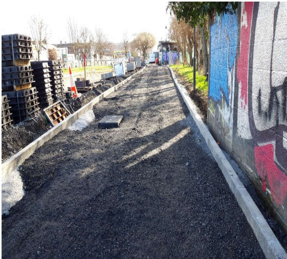
New kerbing works along south & north side towpath – the new kerb delineates the new cycle track and footpath
