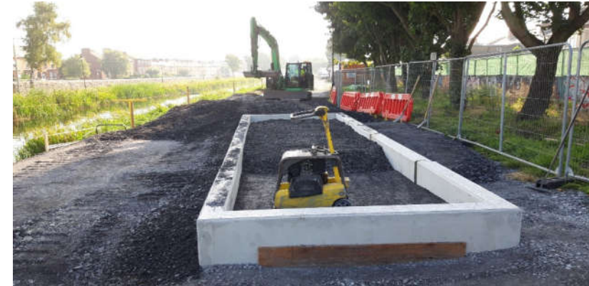
New ESB HV joint bay & ducting
