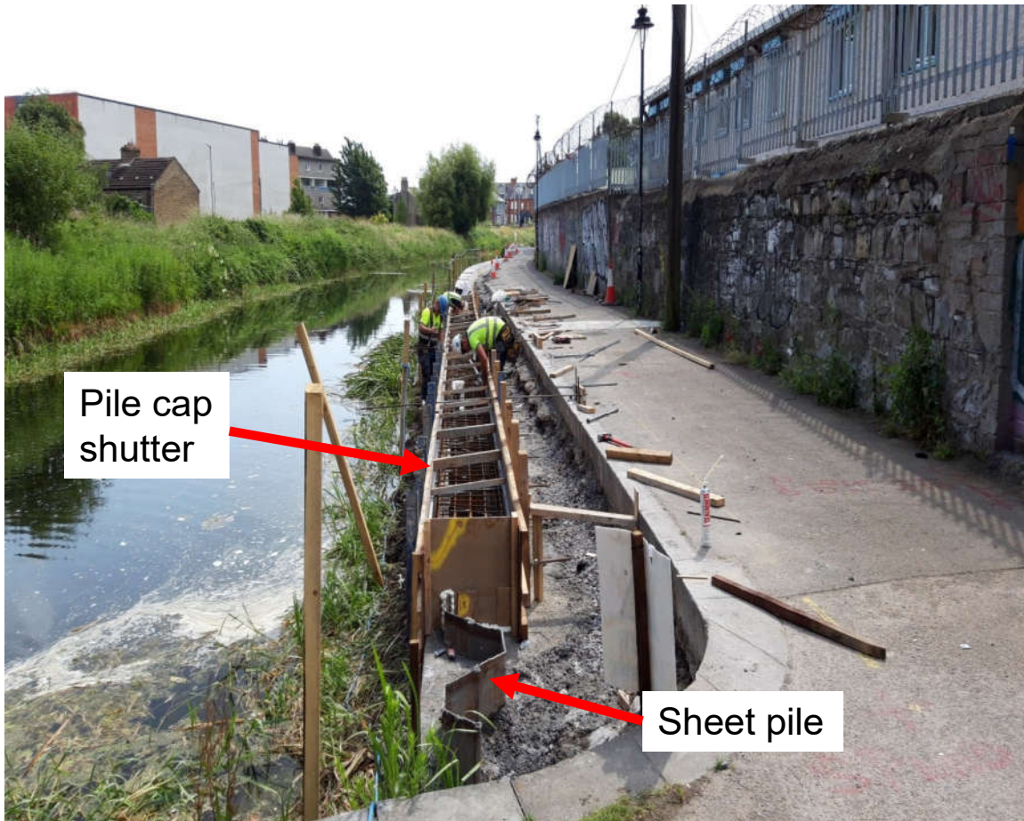
Sheet pile capping beam under construction to widen the footpath / cycle track area
