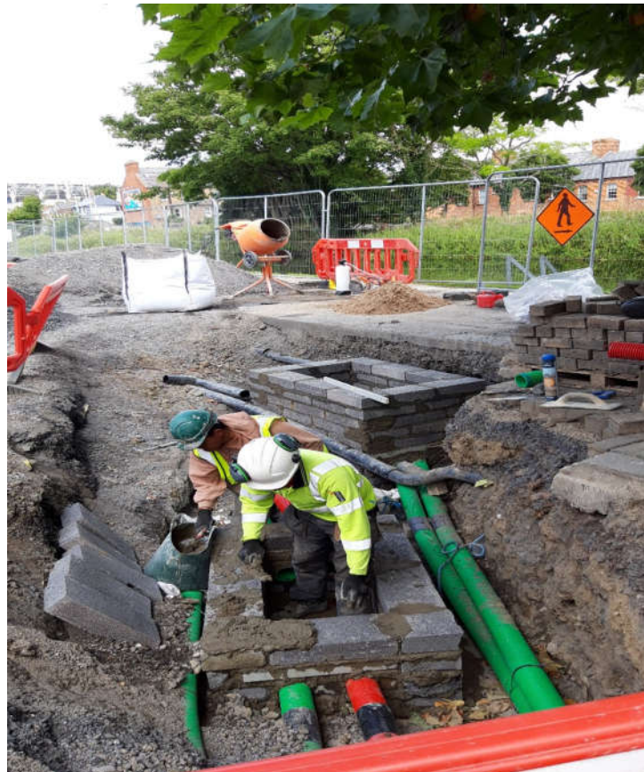
Comms chambers under construction
