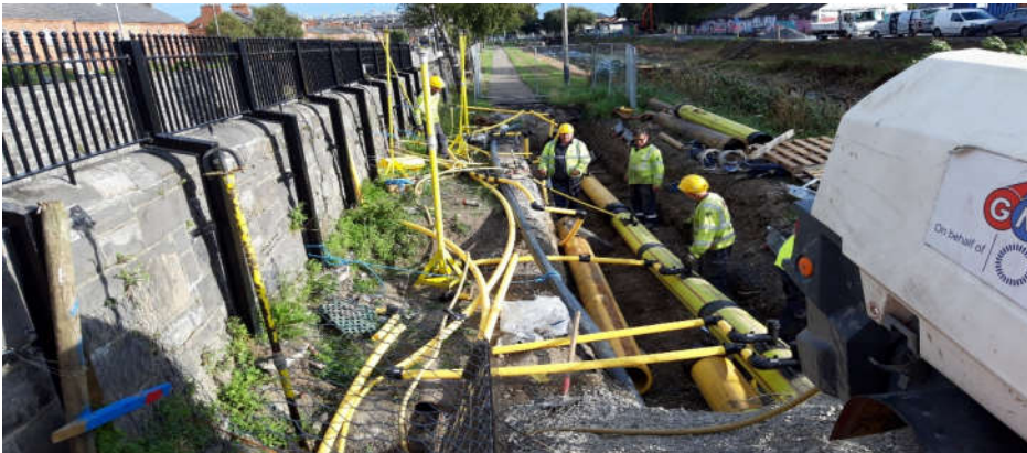
Gas main diversion in north side towpath
