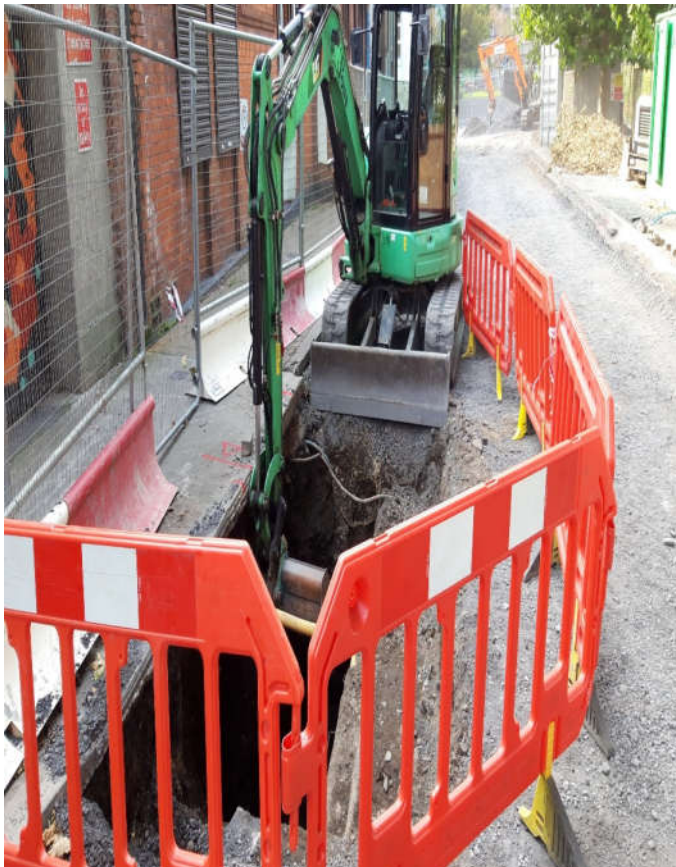
Drainage installation works
