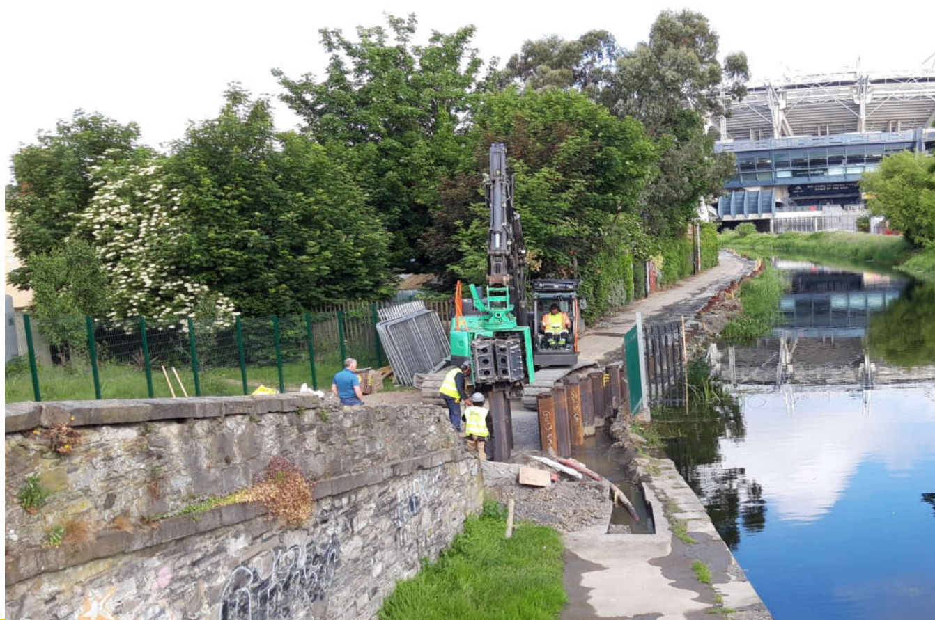
Sheet pile installation works between Bloody Sunday Bridge and Clarke's Bridge west
