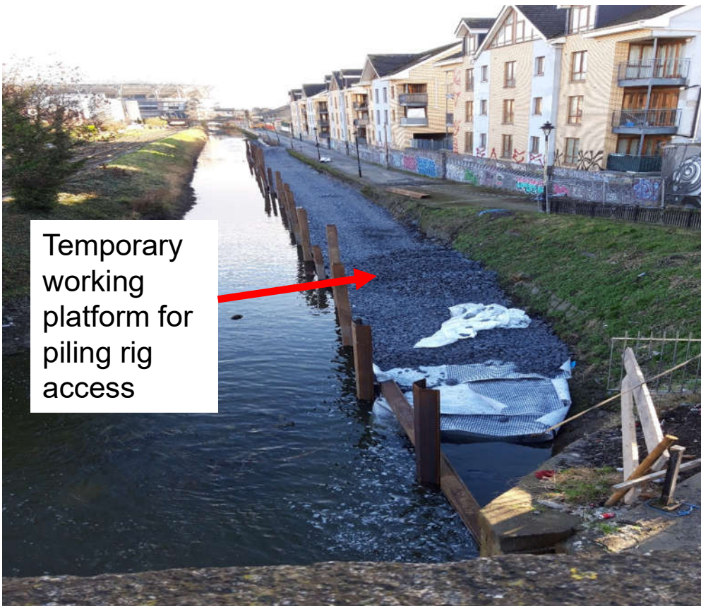
Temporary works platform in canal to facilitate access for the construction of Binns Bridge east side ramp structure
