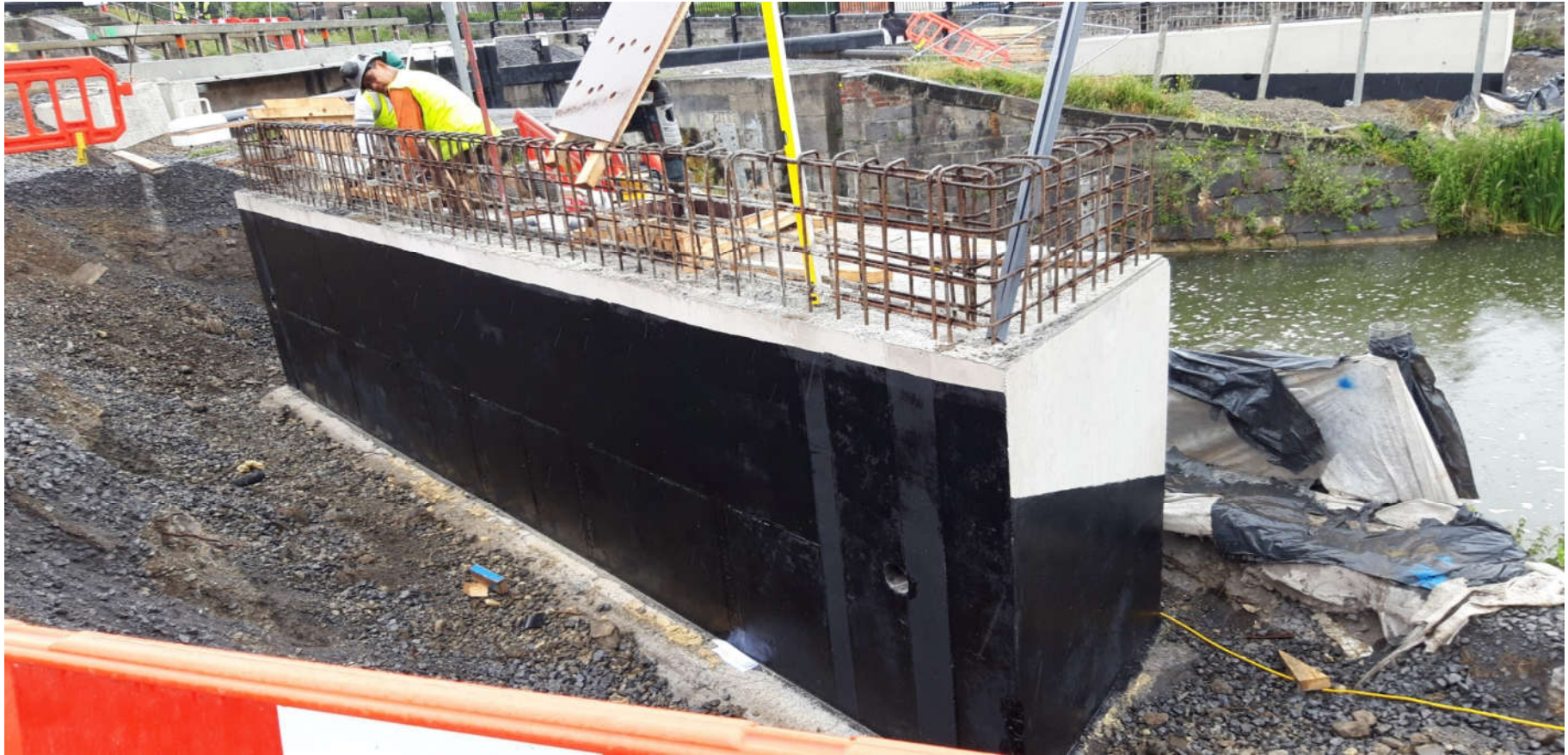
Southside pedestrian bridge abutment construction
