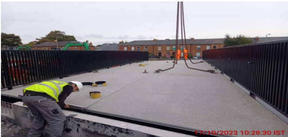
New pedestrian bridge being craned into place adjacent to Lock 3 – October 2023
