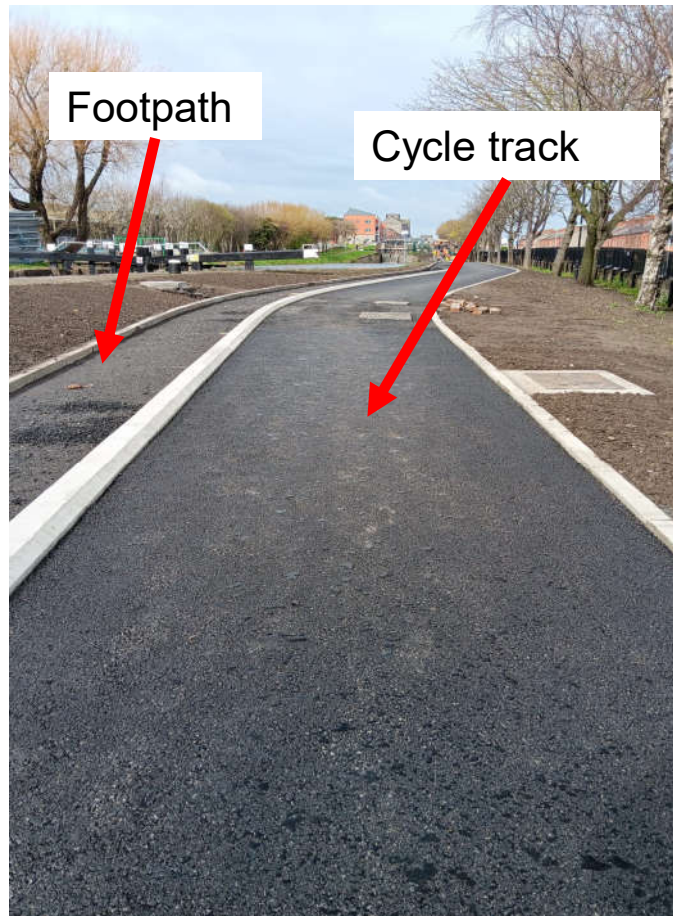
Macadam works along the north side of canal between Cross Guns Bridge and new pedestrian bridge
