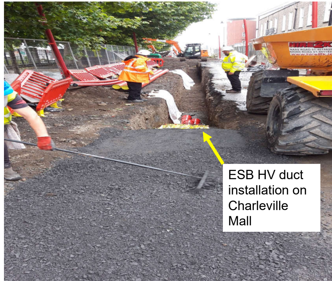
ESB HV duct installation works on Charleville Mall
