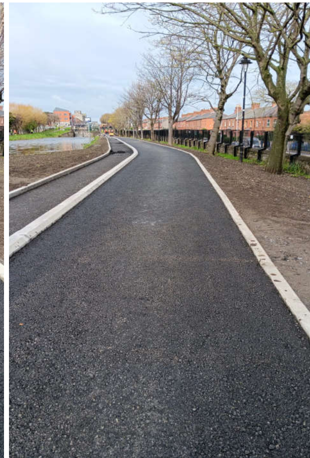
Macadam works along the north side of canal between Cross Guns Bridge and new pedestrian bridge
