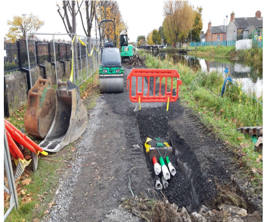
Comms ducting installed along towpath
