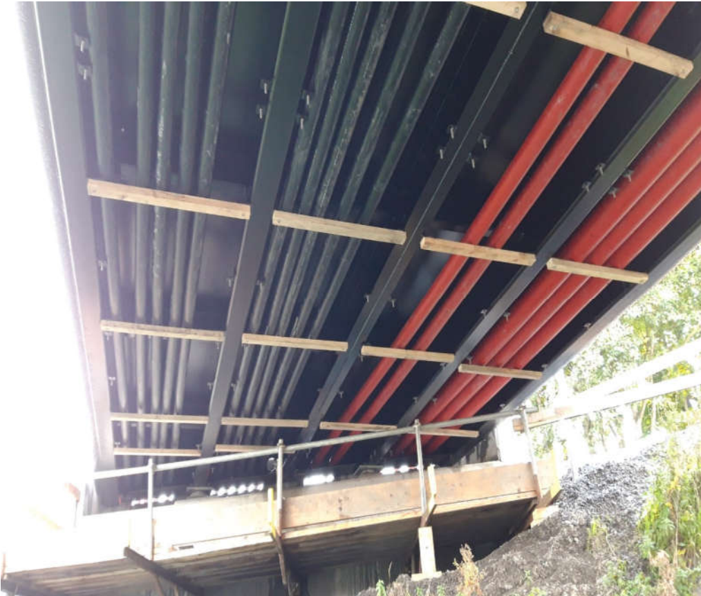
Ducting installed under pedestrian bridge deck
