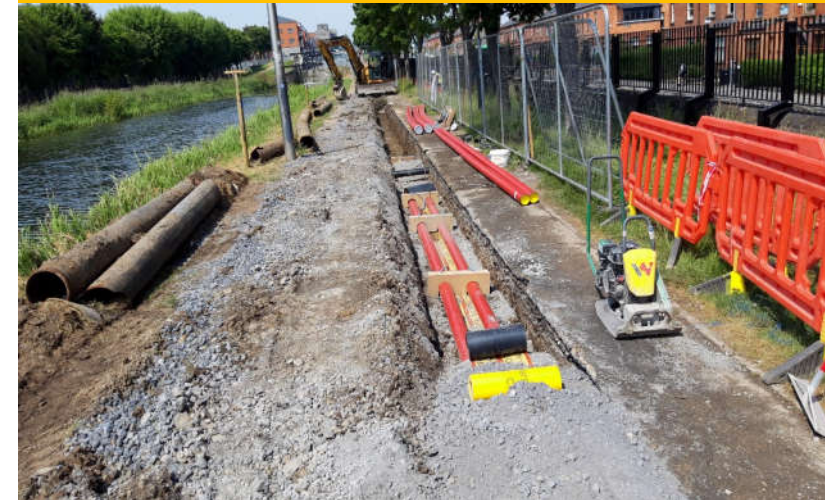
New ESB HV joint bay & ducting
