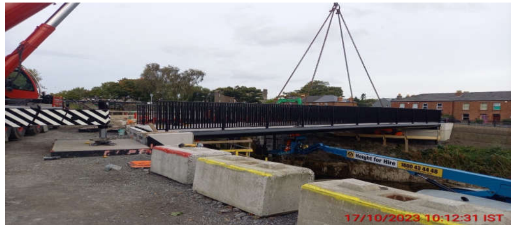
New pedestrian bridge being craned into place adjacent to Lock 3 – October 2023
