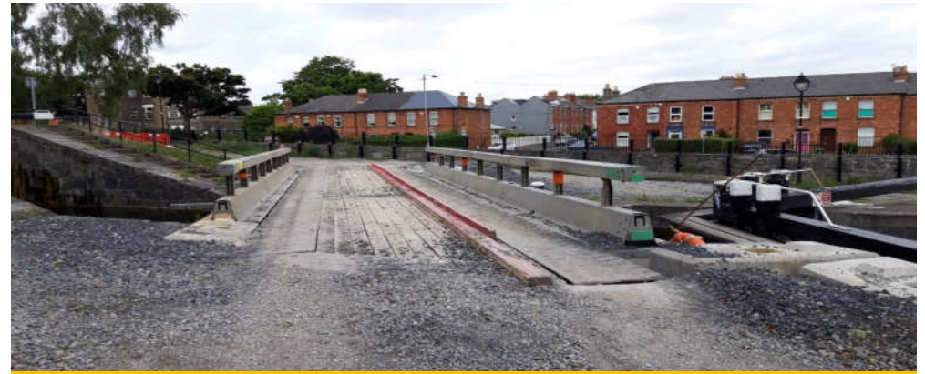
Temporary bridge over canal to facilitate works
