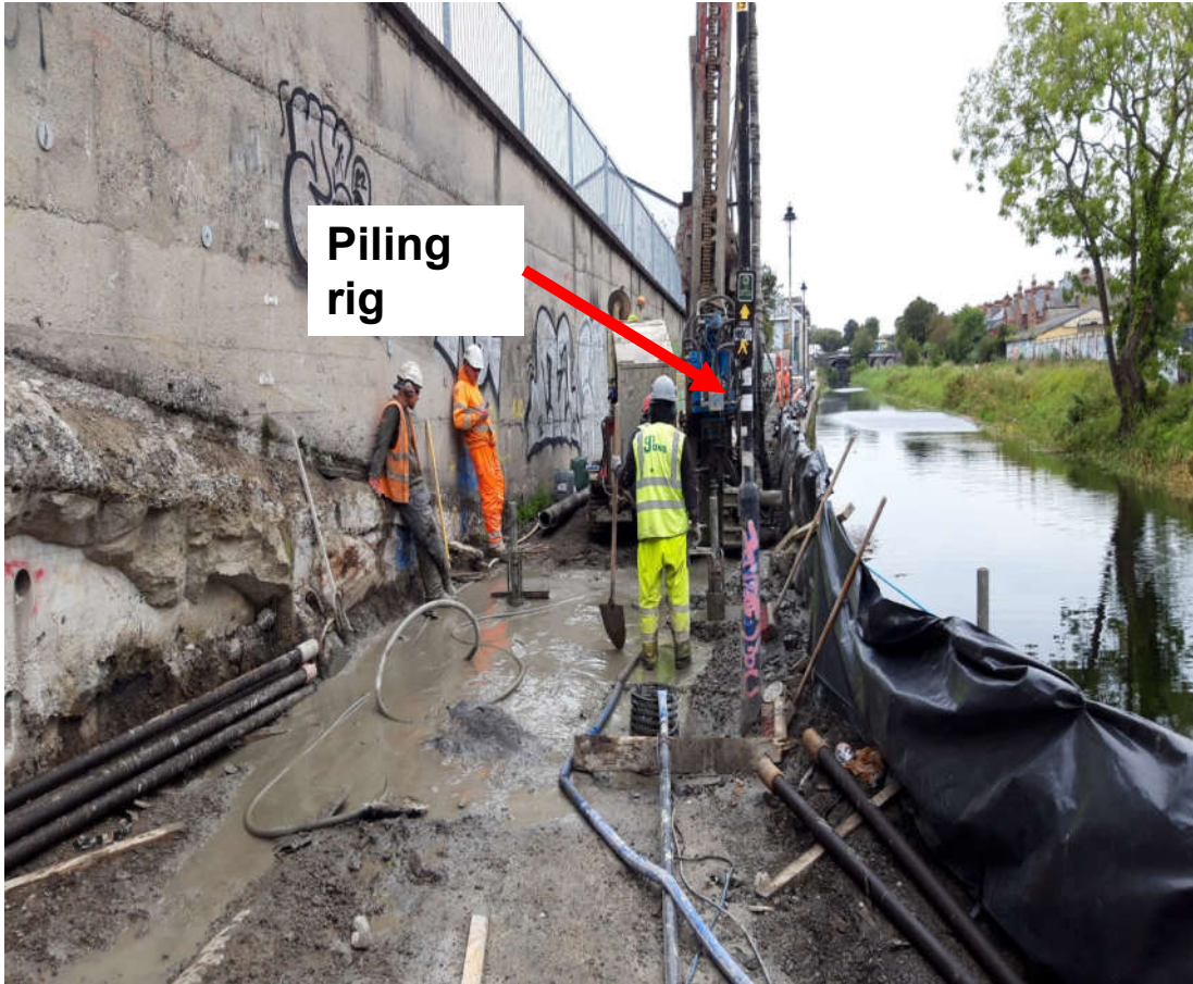
Micro-piling for Russell St. west side ramp structure
