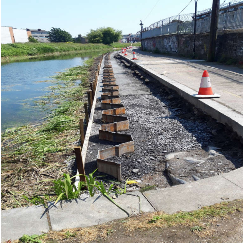
New sheet piles installed between Bloody Sunday Bridge & Clarke's Bridge
