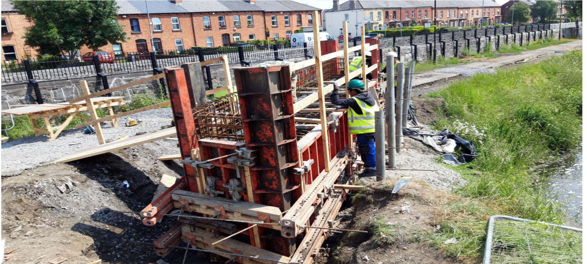
North side pedestrian bridge abutment under construction
