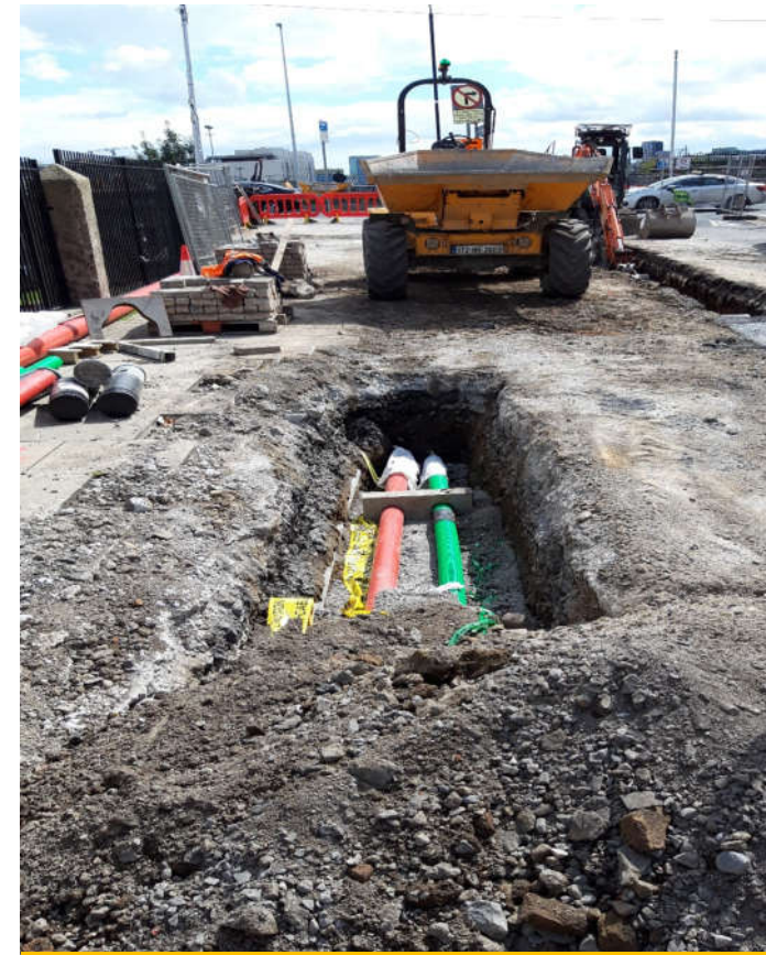
Installing Comms ducting
