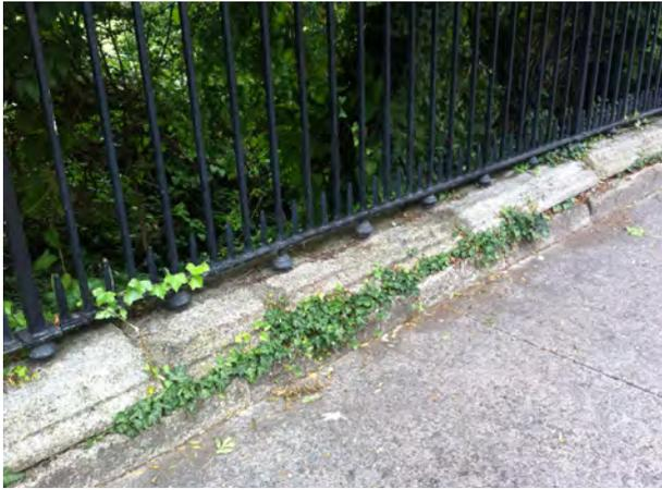
Fig. 73 Detail view of encroachment of ivy causing damage to plinths.
