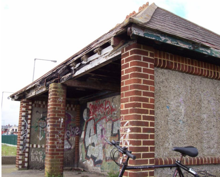
Photo 4.4 Tram Shelter at Dollymount
