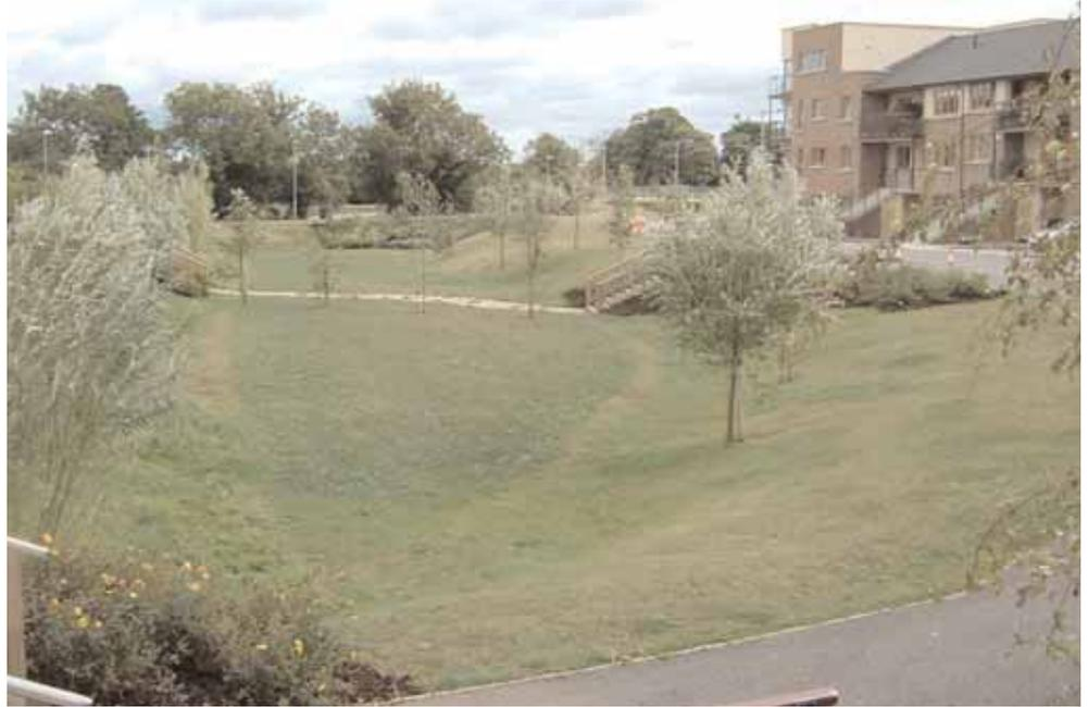
**Photo 3: Detention Basin, Carrickmines - an example of an application of sustainable drainage systems**
