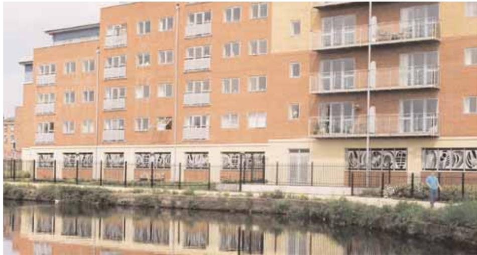
**Photo 6: Habitable floor levels above flood and first floor levels**
