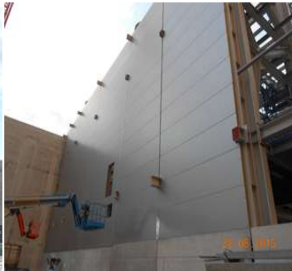
Cladding Turbine Hall (Copyright PML).
