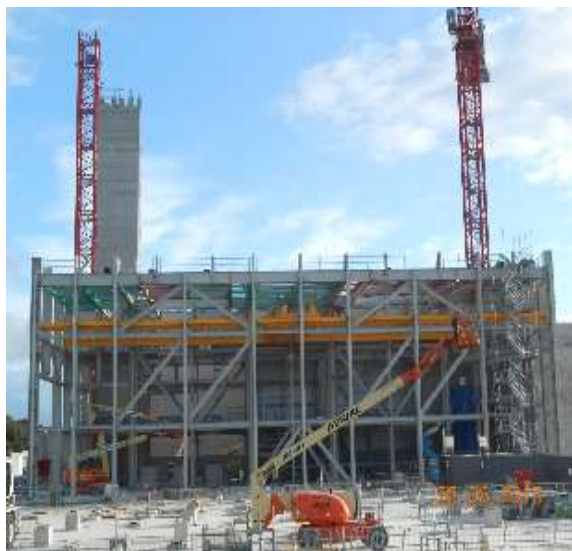
South View of Building Steel (Copyright PML)
