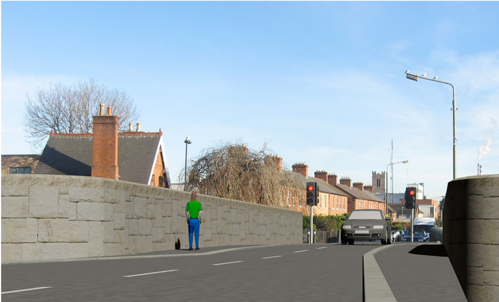
Bridge showing masonry parapet
