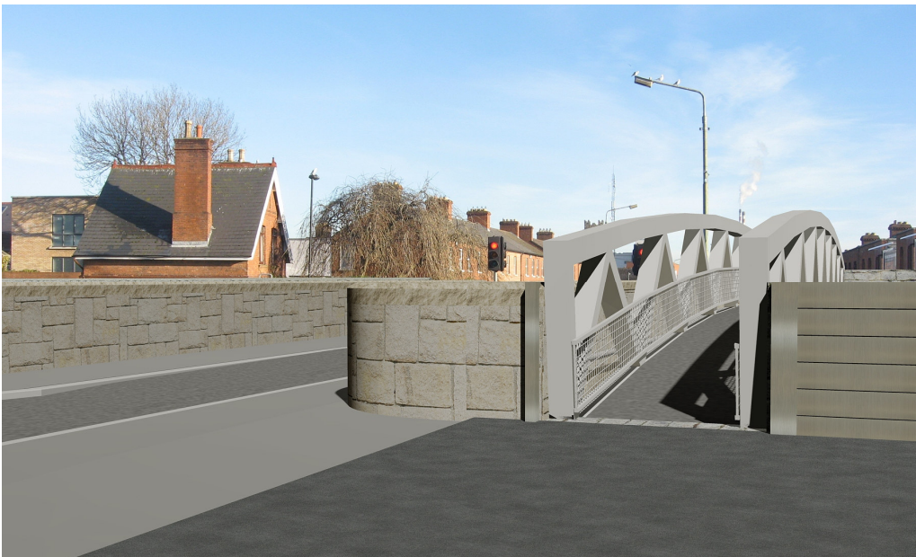
Riverside walkway approach with flood gate in open position
