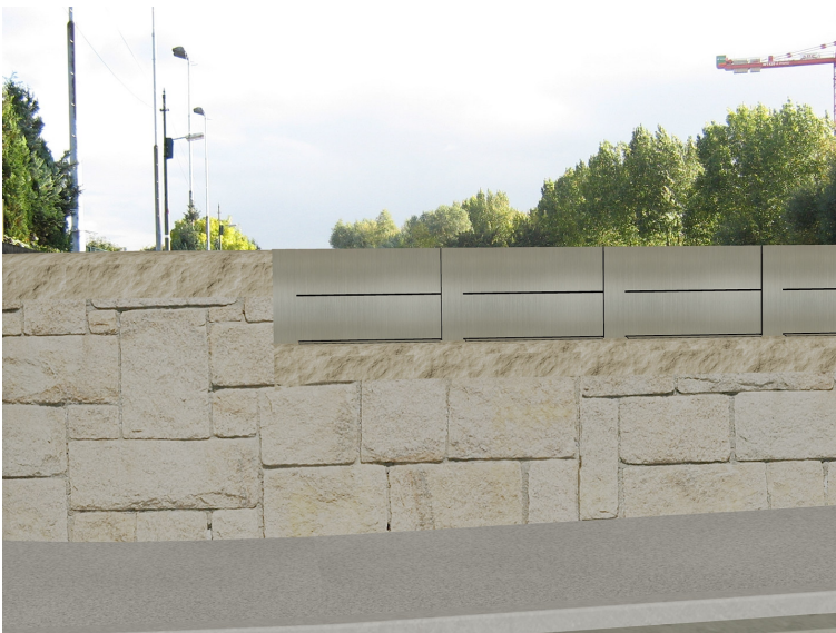
Bridge parapet with emergency demountable defence in place
