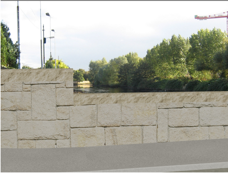
Bridge parapet in normal conditions
