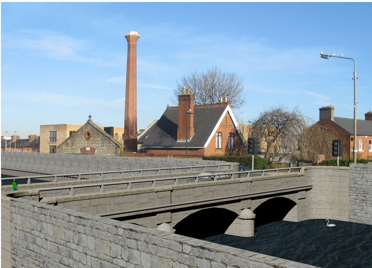
Bridge showing glazed parapet
