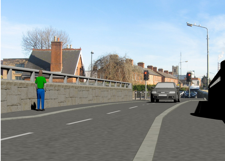
Raised bridge parapet with glazing to allow view
