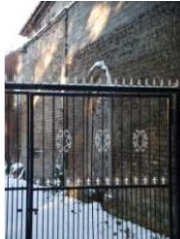
Fine carved stone surround to bricked-up opening in eastern boundary wall
