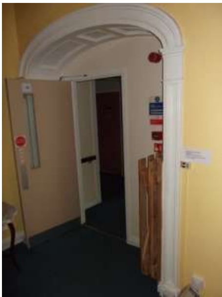
Panelled linings to segmental headed arched opening opening into 'original' cottage off main staircase
