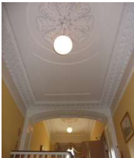
Decorative plasterwork to main staircase
