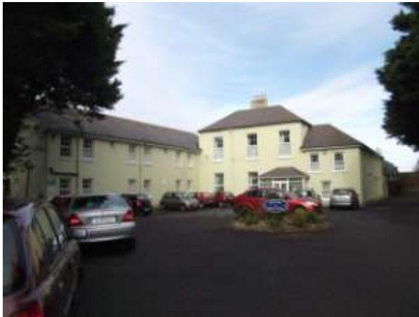
Present entrance elevation with original former thatched cottage on right hand side adjoining the later c1830s three-bay hipped-roofed house in the centre and 1980s extension on the left hand side.
