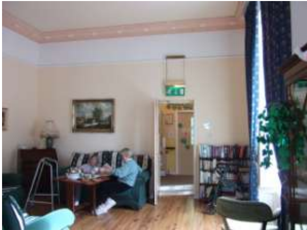
Decorative plaster cornice in ground floor sitting room
