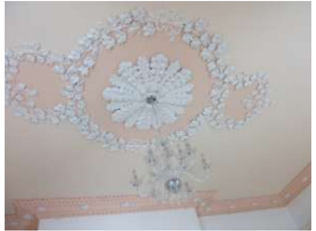
Decorative plaster ceiling rose and garlands in ground floor sitting room
