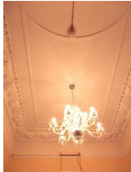
Decorative plaster cornice in front entrance
