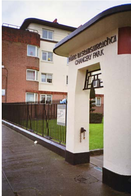
The Chancery Park entrance, photographed by Paul Reynolds as part of Simms120 project documenting the work of Herbert Simms in Dublin.
