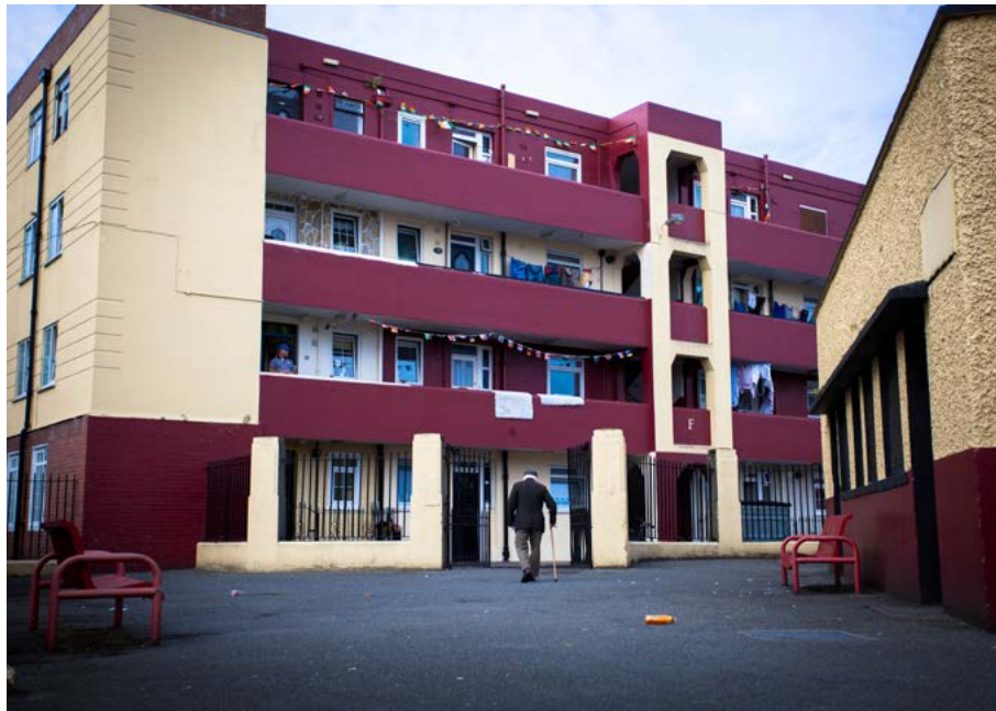
Chancery House flats, photographed by Paul Reynolds as part of Simms120 project documenting the work of Herbert Simms in Dublin
