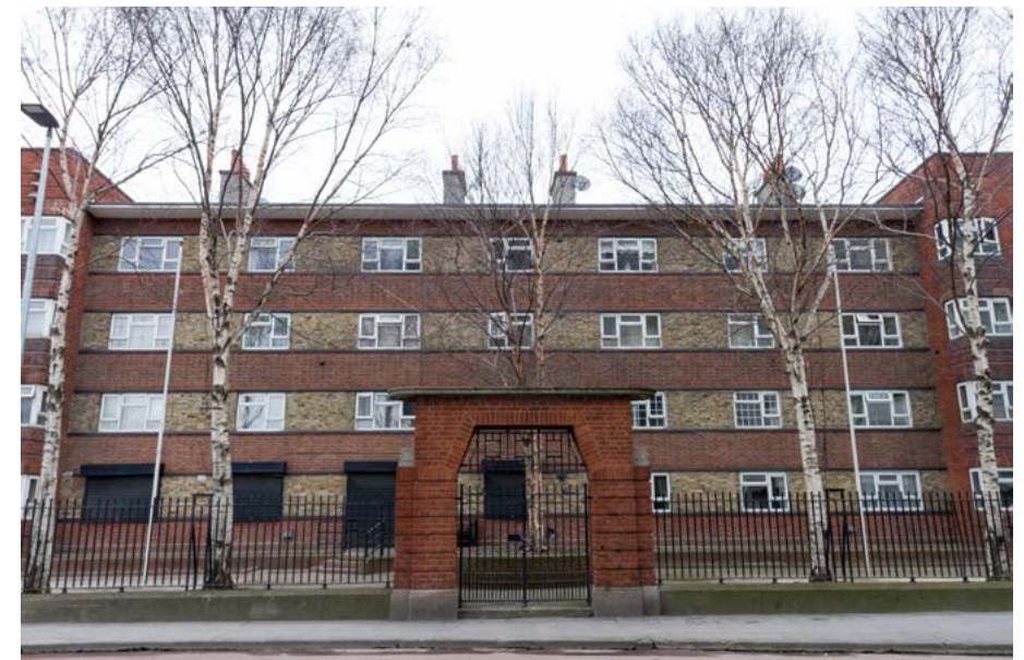
The Marrowbone Lane flats, photographed by Paul Reynolds as part of Simms120 project documenting the work of Herbert Simms in Dublin.
