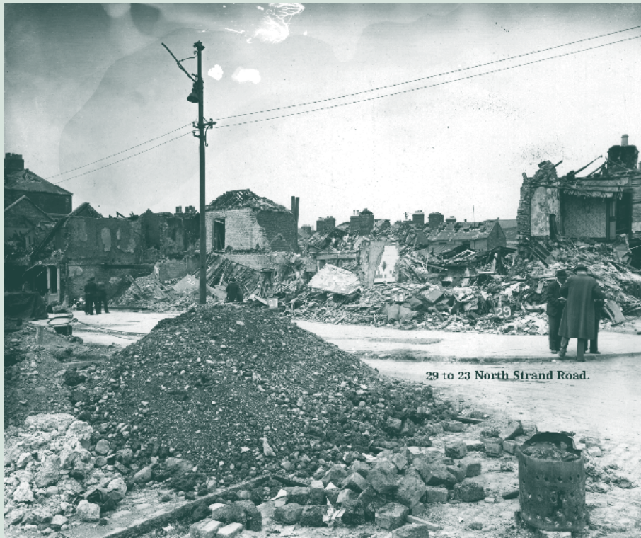
Damage caused by the North Strand Bombing in May 1941 (Courtesy of Dublin City Library and Archives)
