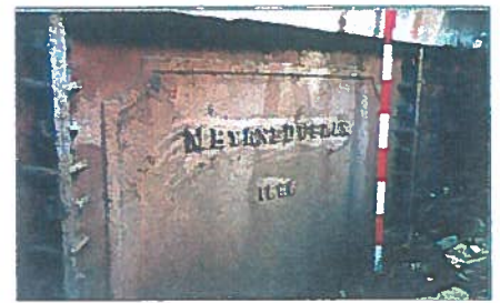
A panel of the cast-iron sectional aquaduct
