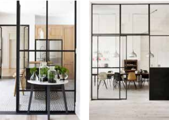
Figure 6. Steel and glass partitions in historic residential scheme. It can be difficult to achieve the slim profiles shown where partitions require to be fire-rated. (source: www.koldby.com & www.trendecora.com)
