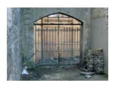
Fig. 7.9 Inner, rendered face of Newmarket entrance gate prior to temporary removal of gate and propping with concrete blockwork.
