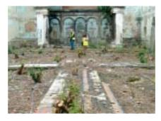
Fig. 7.28 Detail view of tiled aisle. Growth, although cleared recently, still persists and has taken root in brick structure.
