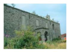
Fig. 7.13 North (front) façade showing vegetation at wall tops and generally loss of mortar in joints with detail of bellcote below, showing loose stone and open joints. The bell, which was cast in 1903, from the two original bells of 1714, is now displayed in St. Patrick's Cathedral.
