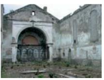
Fig. 7.15 Internal view of church, showing considerable amount of internal plaster surviving, the east end chancel and the scar where the dado panelling was removed.
