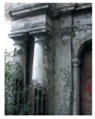
Fig. 10.6 The fine and relatively intact Classically inspired east chancel remodelled and extended in 1899-1900. The unusual construction of the double pilaster Tuscan columns is notable.
