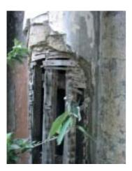
Fig. 1.3 The classical plasterwork in the chancel is in a state of decay.
