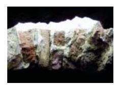
Fig. 7.27 View through ope in floor showing brick vault construction to crypts.
