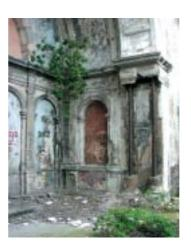
Fig. 7.17 View of south double pilaster where iron column structure has been completely exposed.
