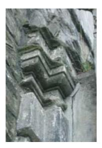
Fig. 7.22 Awkward detail of junction between early granite door surround on north façade and later Victorian porch. Note traces of surface decoration on granite in addition to loss of detail and surface delamination of stone.
