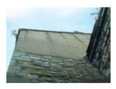
Fig. 7.14 Section of dense cement render on the east gable with some cement pointing under – probably date to early 20th century construction of apse.
