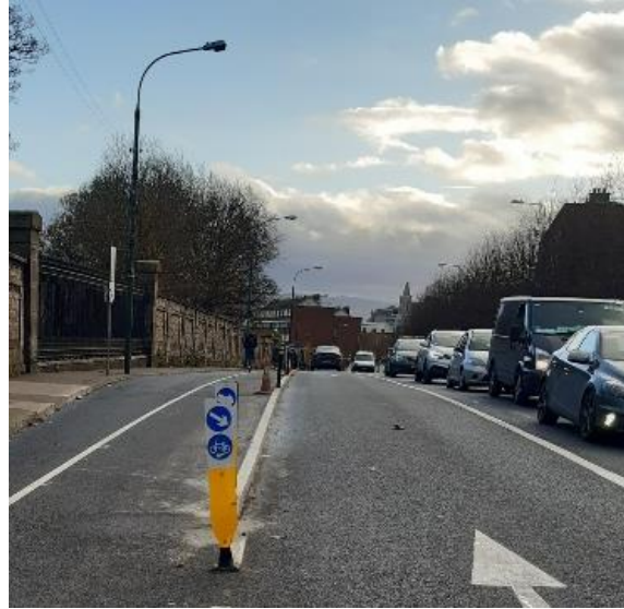
Extruded kerb outbound and inbound on Constitution Hill
