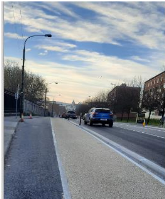
Extruded kerb with bollards and buff surfacing on Constitution Hill
