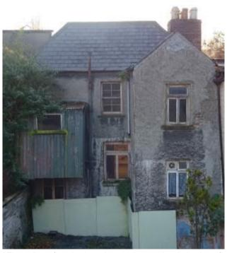
Fig.6: Rear/north elevation with steeply pitched roof and gabled closet return (indicative of an early date).
