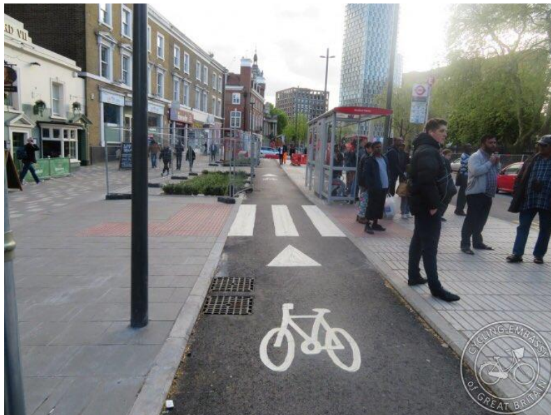
Figure 5. Photograph of an Island Bus Stop in London, with a one-way black asphalt cycle track running between a concrete paved pedestrian area and a bus stop island with bus shelter. Two crossings are provided, one on either side of the bus shelter, with the black asphalt cycle track ramping up to footpath level at the crossings. There is zebra painting on the asphalt cycle track at the crossing, and there is L-shaped red tactile paving on the footpath on either side of the cycle track.
