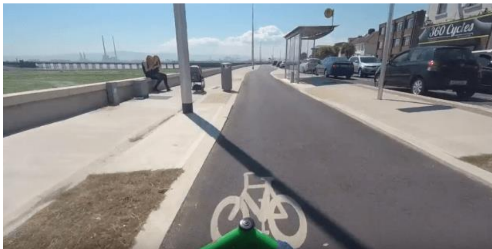
Figure 4. Photograph of the Sutton to Sandycove Cycle Track, with a concrete Bus Island at the front of the footpath, and a black asphalt, two-way cycle track running between the footpath and the Bus Island. Two crossing areas are provided, one in advance of the bus shelter, and one past the bus shelter. At the crossings the footpath dishes down to the level of the cycle track and rectangular, buff-coloured tactile paving is provided on the footpath on either side of the crossing. No guidance tactile is provided.
