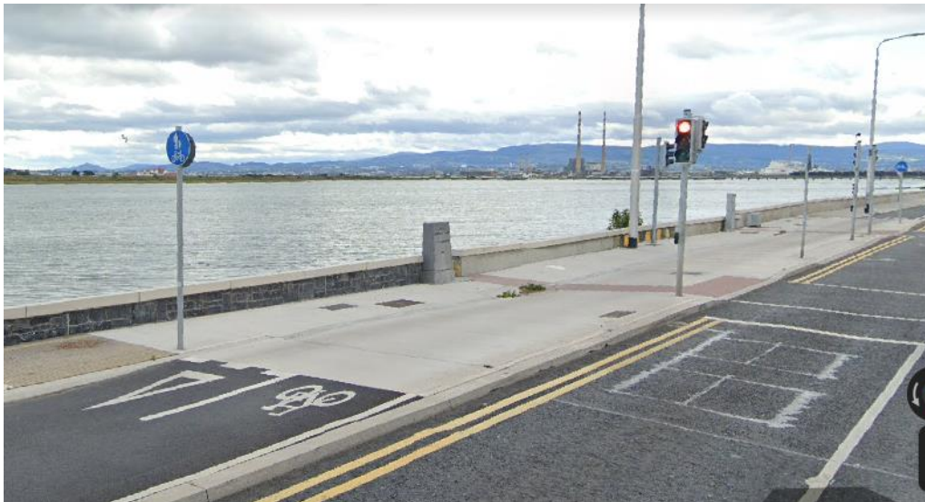
Figure 7. Photograph of the Sutton to Sandycove Cycle Route: A two-way cycle track runs parallel to a footpath, with the footpath on the inside and adjacent to the sea wall. The cycle track terminates in advance of a signalised pedestrian crossing, creating a shared space. The cycle track is black asphalt and ramps up to footpath level at the start of the shared space. A shared space sign is mounted on a pole on the footpath at the end of the cycle track. Ladder tactile paving is in place at the start of the concrete footpath adjacent to the cycle track. No tramline tactile is in place at the start of the cycle track.
