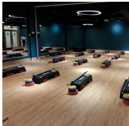
Construction of Multi-Purpose Studio in SPORTSCO.
