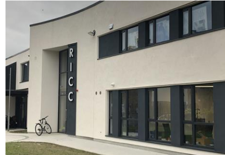
Refurbishment of Ringsend and Irishtown Community Centre.
