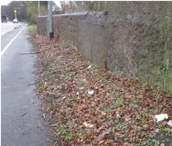
Figure 3.52 Mass concrete wall at west end
