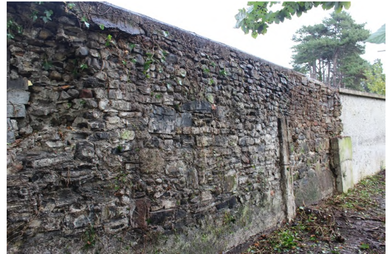
Figure 16 Section with Slight Bulge (Inner Face)
