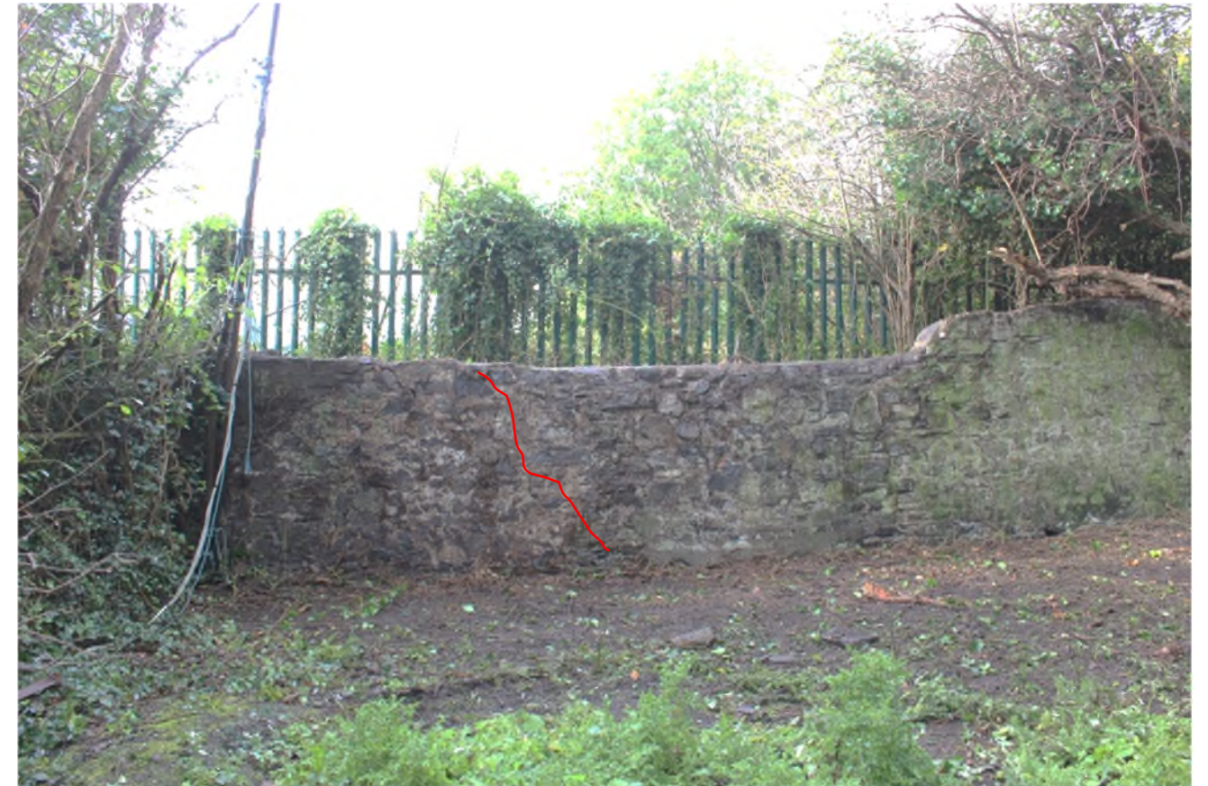
Figure 18 West Boundary Wall - Typical Crack Highlighted in Red
