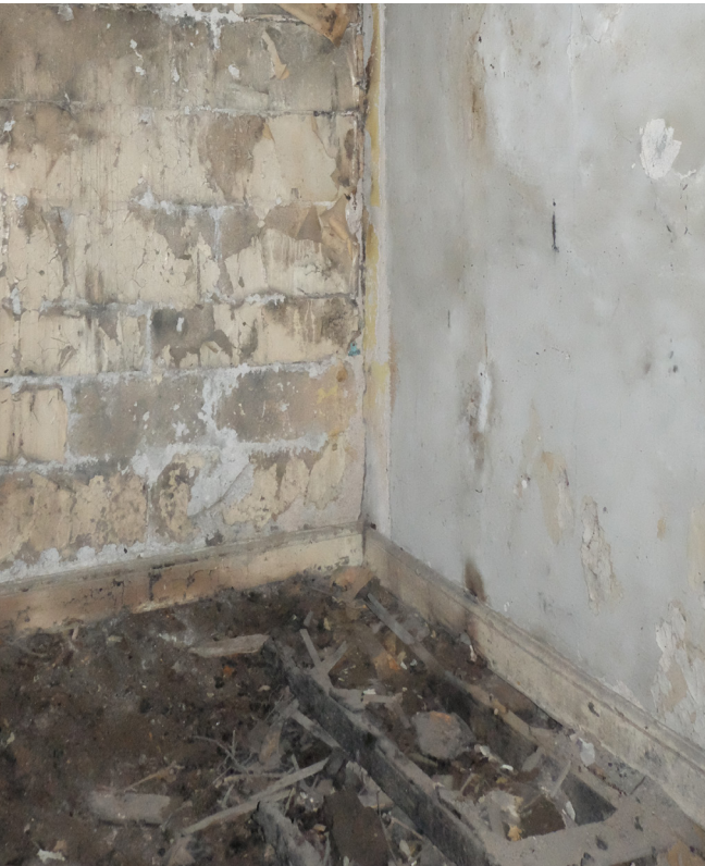
Figure 3.22 Decayed suspended timber floor in north west corner of Room18-02
