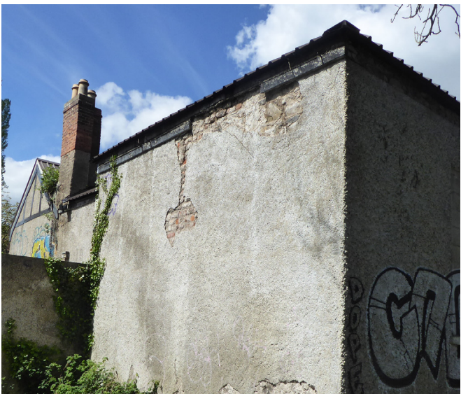
Figure 3.04 Eaves detail of 19th century east wing. Brick of chimney constructioun visible in the wall
