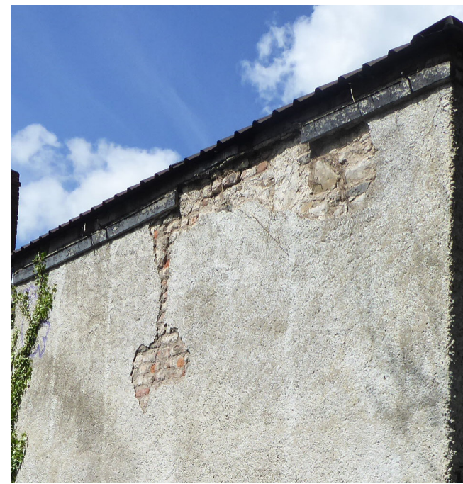
Figure 3.09 Brickwork to 19th century chimney visible through failed render on south elevation of 19th century east wing.
