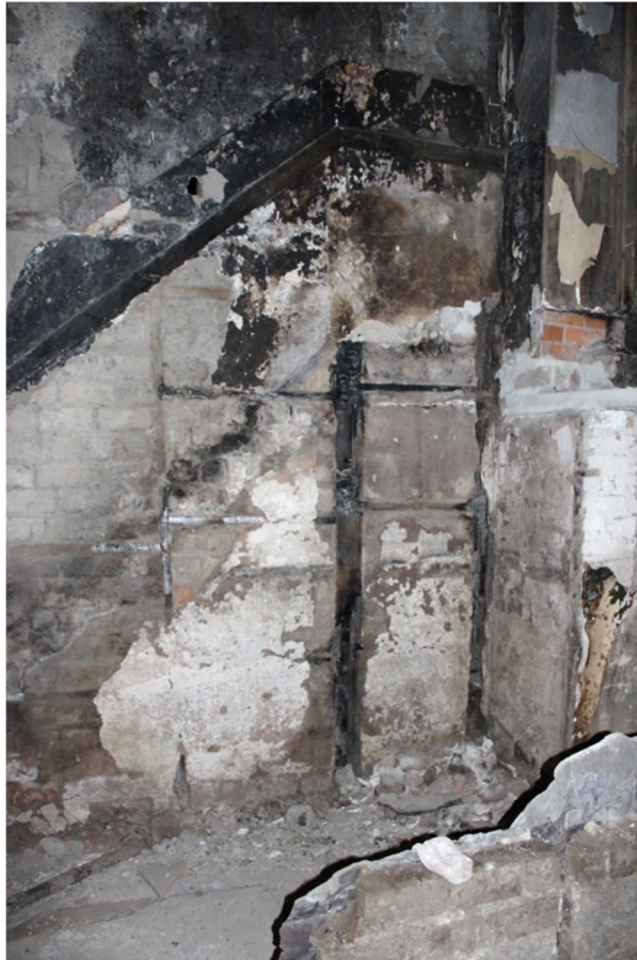
Figure 6 Fire-Damaged Internal Partition
