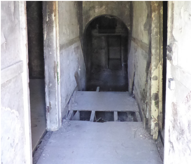
Figure 3.24 Suspended timber floor to room 19-06, with unstable joists and missing boards.
