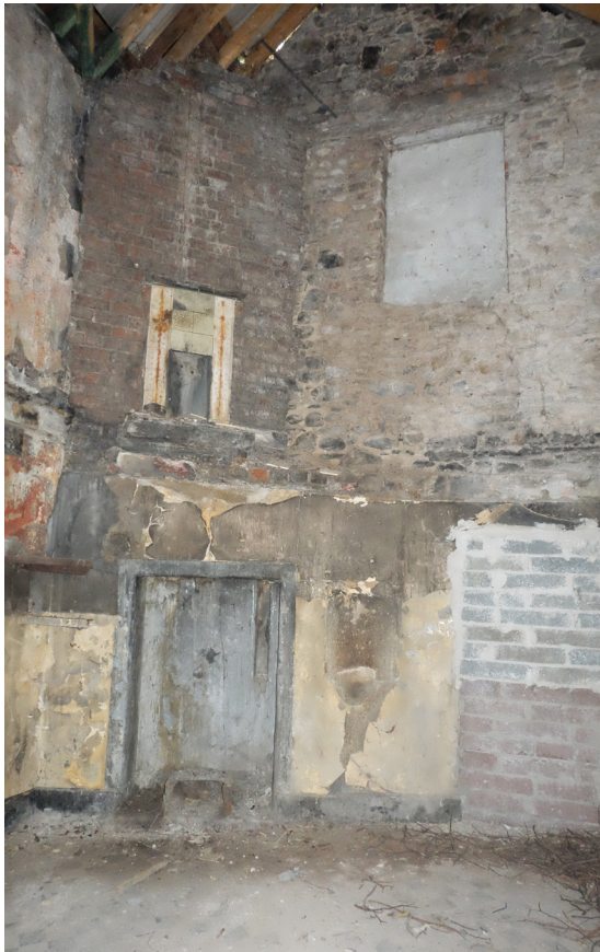
Figure 2.21 Southeast corner 20th C tiled fireplace at upper level, earlier fireplace at ground floor level
