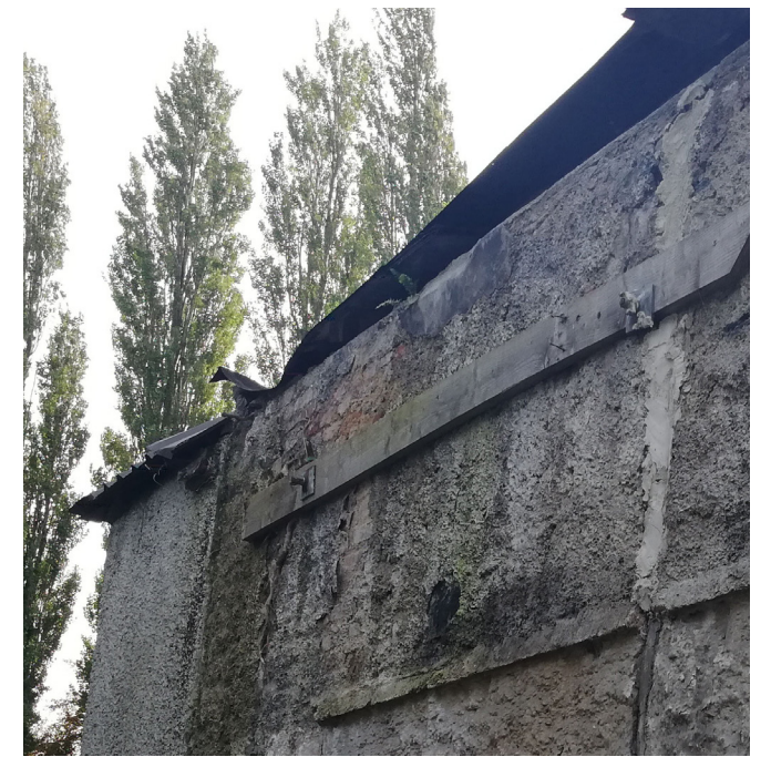
Figure 3.10 Brickwork to 19th century chimney visible through failed render on north elevation of 19th century east wing
