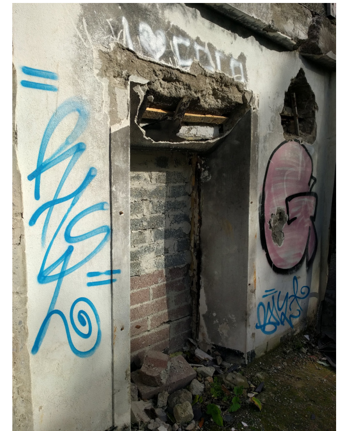
Figure 3.16 South Elevation 18th C wings More evidence of reinforced steel embedded within the concrete on south elevation.
