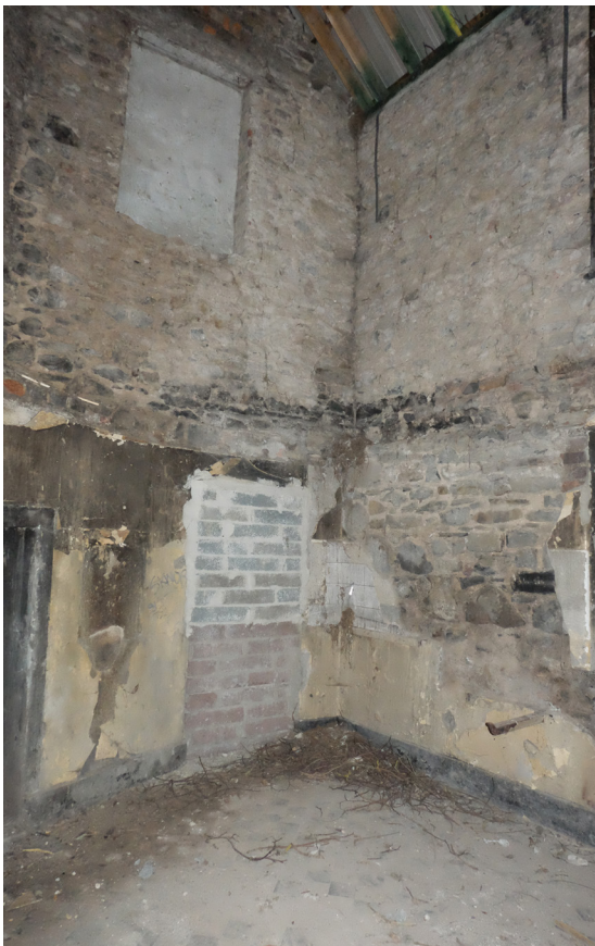
Figure 2.22 Southwest corner Blocked former doorway into single storey extension
