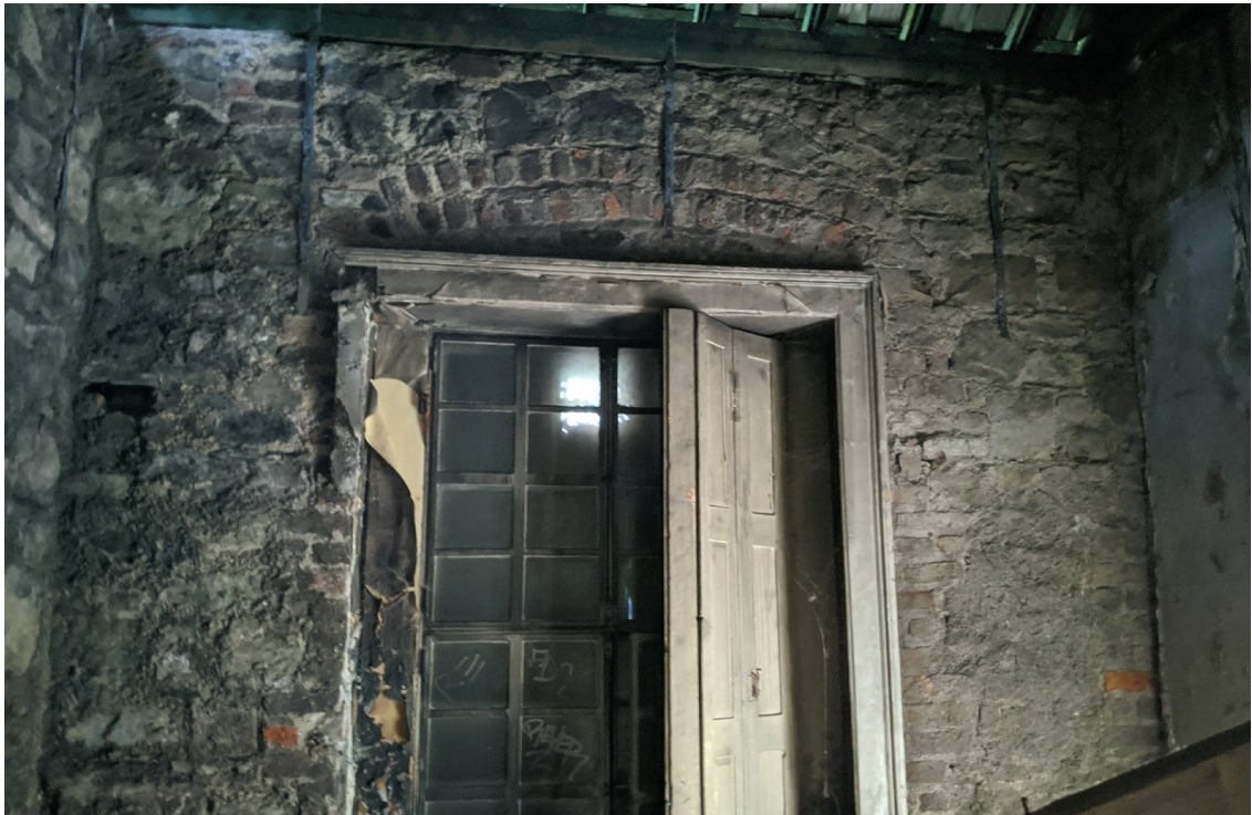
Figure 2.40 Room 19-07 Window (East wall) Brick relieving arch, surviving shutters, windows and steel secondary glazing
