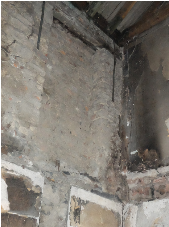
Figure 2.25 Northwest corner Brick recess in west wall.
