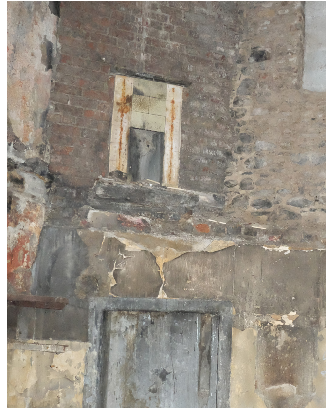
Figure 3.29 Room 18-01: note different angle, and lack of bonding of upper chimney breast.
