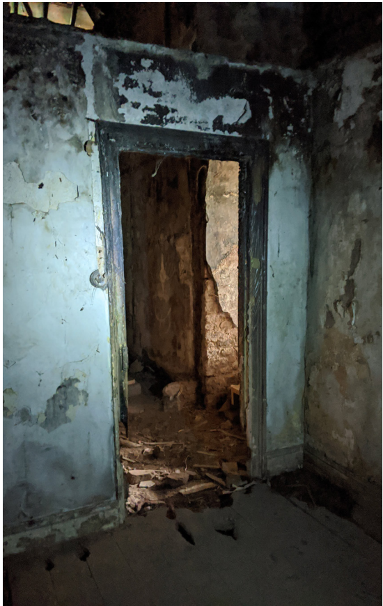
Figure 2.31 Northwest corner Surviving architrave to door, looking into Room 18-03.
