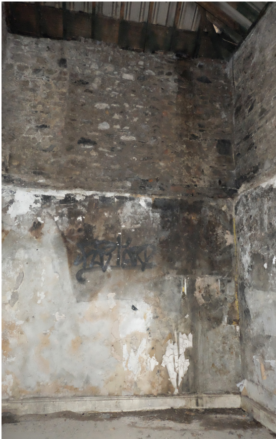
Figure 2.27 East wall Plaster, timber floor and skirtings survive at ground floor
