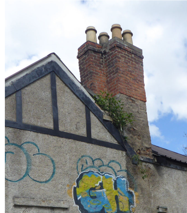
Figure 3.07 Double chimney stacks on south elevation serving the 18th century wings of the building.
