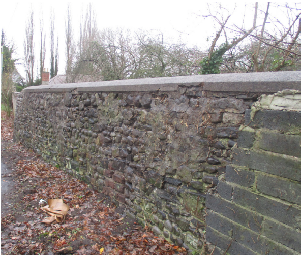
Figure 3.51 Stone wall at east end, Note the blockwork repair
