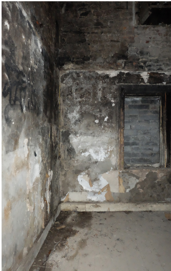
Figure 2.28 Southeast corner Architrave to window survives, but damaged by fire
