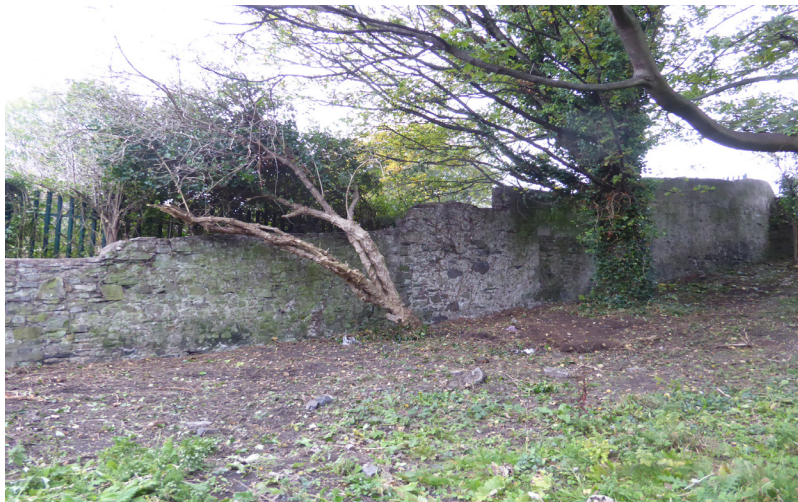
Figure 3.59 The stone western boundary wall follows the slope of the land. The blocked doorway is beside the sycamore tree.
