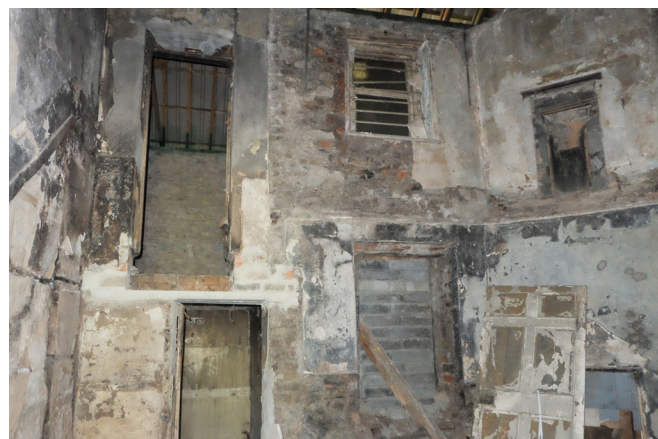
Fig. 2.15 The interior of the central, 18th century wing. All the upper floor structure has been lost, but fireplaces and a two storey partition survive.
