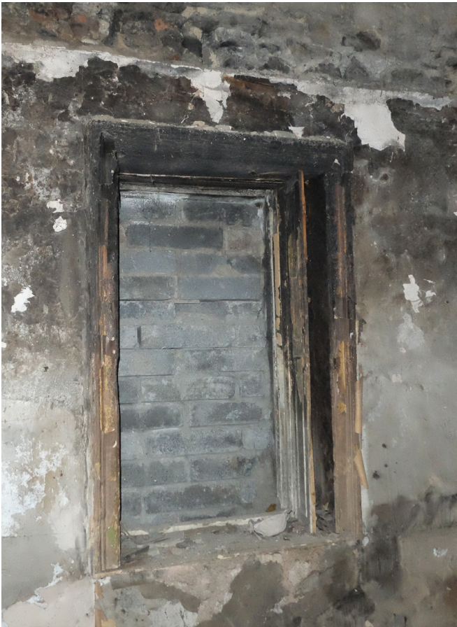
Figure 3.39 Fire damaged timber architraves & reveals. Room 18-02
