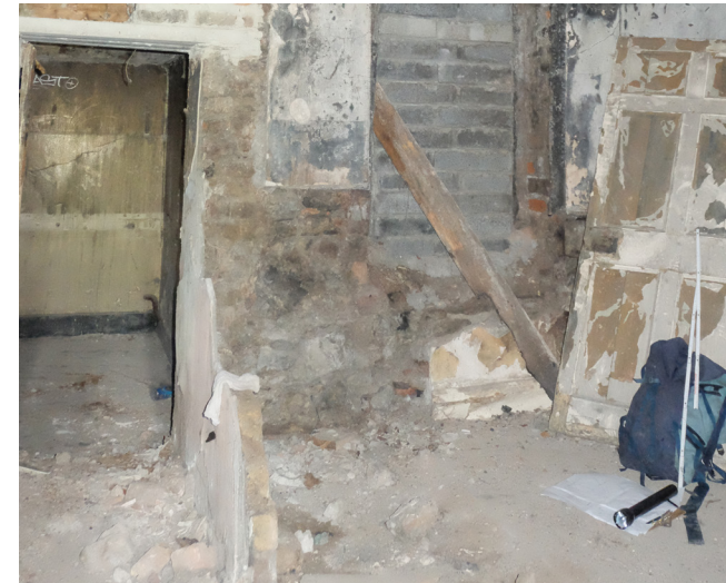
Figure 3.18 Remains of lost partition to the hallway between rooms 18-03 & 18-04.
