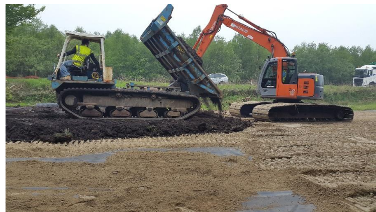
Depositing contaminated Japanese knotweed soil in bund
