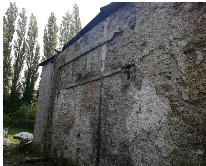
Figure 3.11 North elevation Large open joint between 18thC and 19thC phases of build. Sockets for former floor structures.
