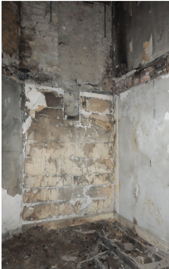
Figure 2.30 Northwest corner: Partition wall to right. Damaged timber floor
