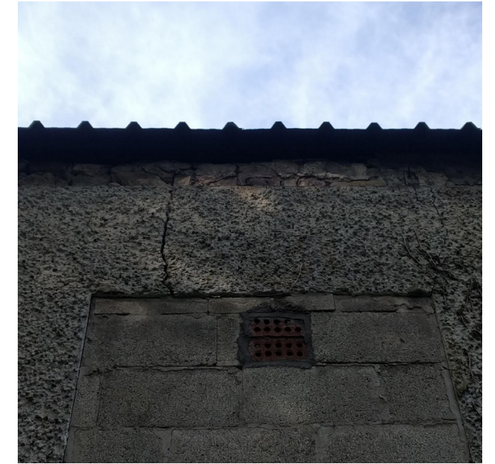
Figure 3.14 East Elevation Crack at the window head at the east elevation of the 19th century wing.
