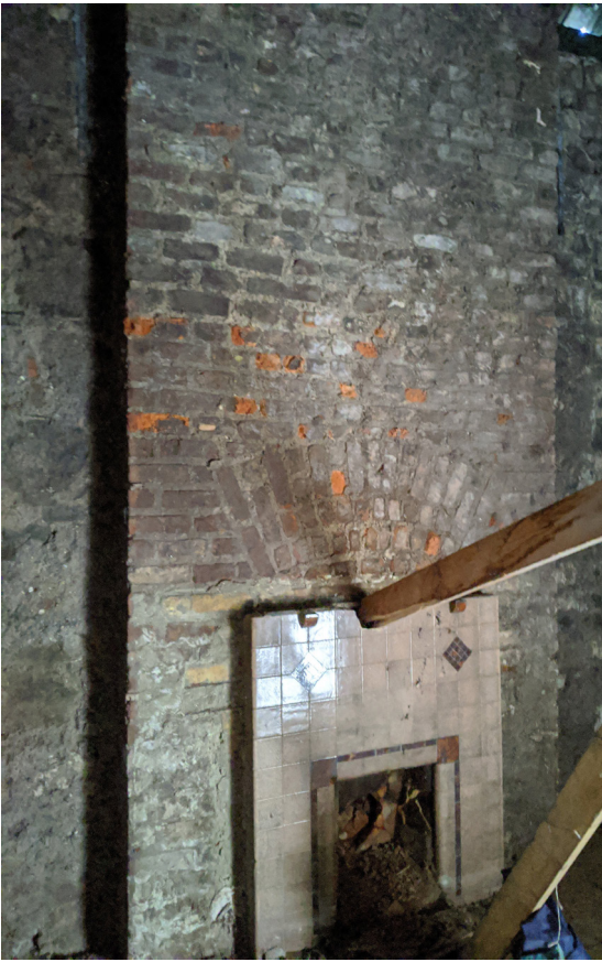
Figure 2.44 North wall: 20th C tiled fireplace. Brick chimney breast bonded into wall
