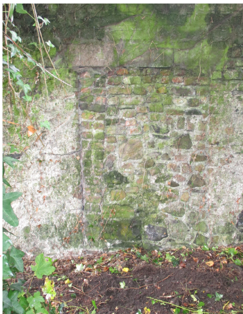
Figure 3.66 Bricked up doorway in west boundary wall
