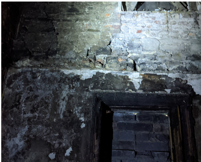
Figure 3.26 Pockets in stone wall of 18-02 shows direction of joists and level of upper floor.
