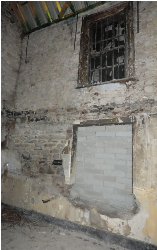
Figure 2.23 West wall: six over six sash window, security bars and architraves survive at the upper floor
