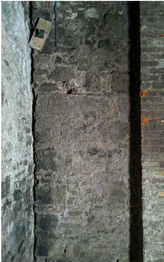
Figure 2.43 Northwest corner Open joint at junction between 19th and 18th C walls
