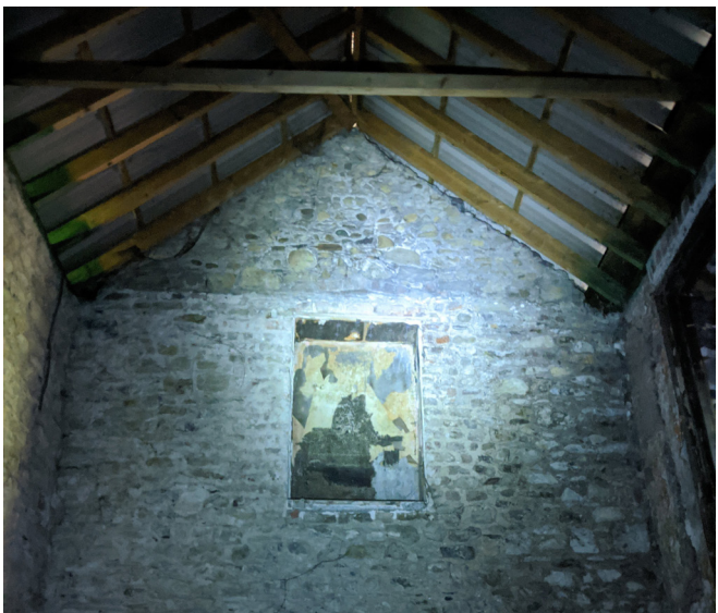
Figure 3.03 North gable of the 18th century west wing; possible construction joint
