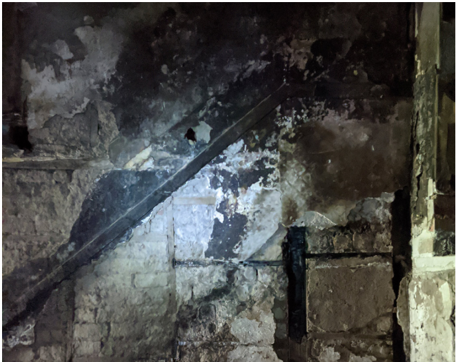
Figure 3.41 Traces of stair and handrail on partition wall between 18-03 and 18-02.
