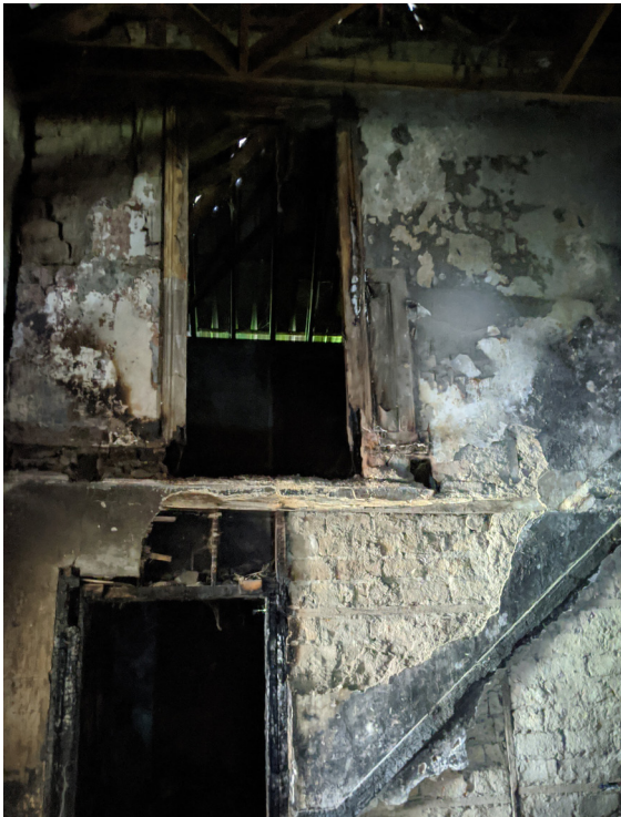
Figure 2.33 - 34 South Wall: Brick partition with timber noggins. Line of handrail and stair stringer visible. The timber base plate of this wall is rotten and the structure fragile.
