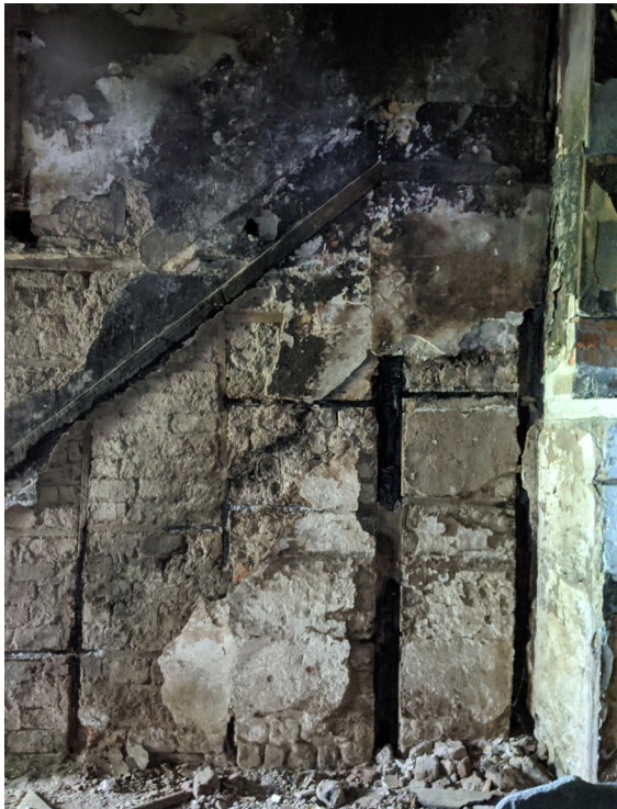
Figure 2.33 - 34 South Wall: Brick partition with timber noggins. Line of handrail and stair stringer visible. The timber base plate of this wall is rotten and the structure fragile.
