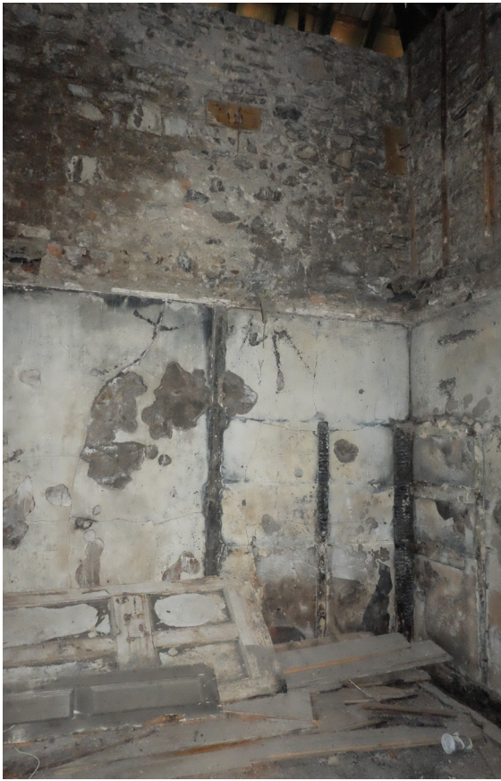
Figure 2.37 Northeast corner Remains of partitioned space indicated by timbers in wall. Salvaged doors, shutters and boards.
