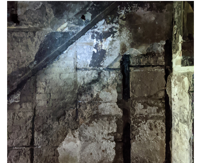
Figure 3.19 Surviving brick nogging partition displaying charred timbers and scar from stair
