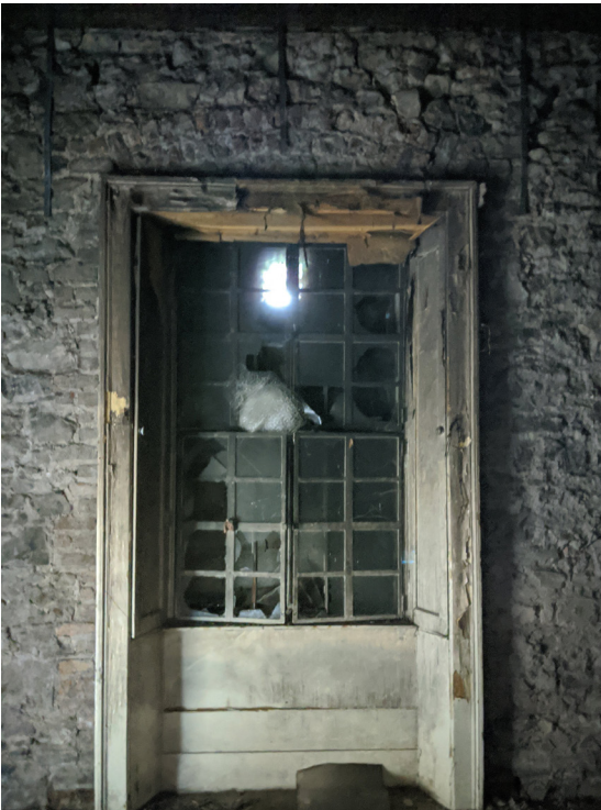
Figure 2.50 East Wall: Sash window, architraves, shutters and steel secondary glazing
