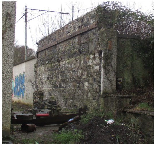
Figure 3.63 Calp stone wall at north side of the house. Low retaining wall to drive in foreground. Tram gantry beyond
