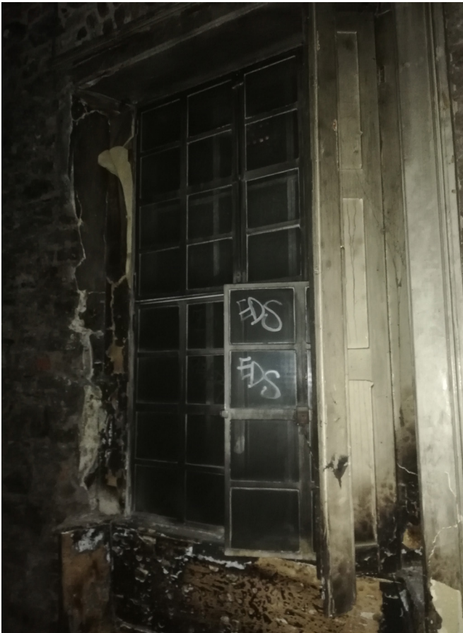
Figure 3.34 Sash window, timber shutters, and steel secondary glazing Room 19-07
