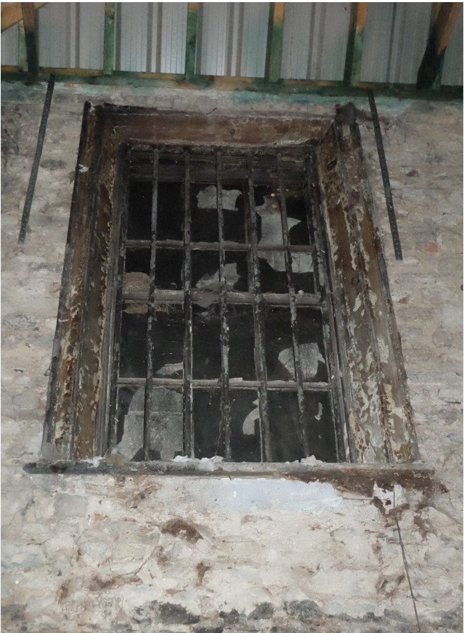
Figure 3.38 Sash window, timber architraves, reveals & window board, iron bars. Room 18-01
