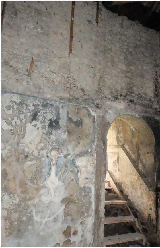
Figure 2.38 East wall: arched opening into 19th century wing. Smooth plaster indicates extent of former corridor 18-03 .
