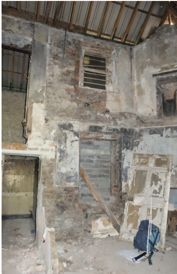
Figure 2.35 West wall Remains of former partition wall to Room 18-03 beside doorway into Room 18-01 .
