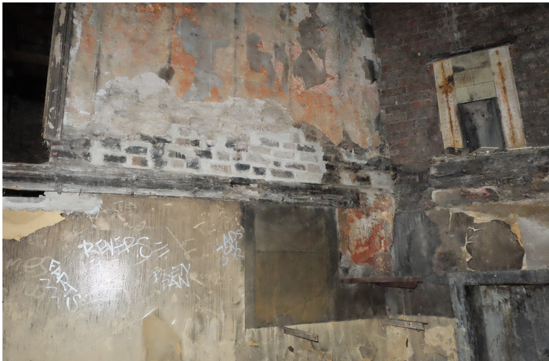
Figure 2.17 Southeast corner See scars of repairs and alterations. Brick chimney breast at upper floor is not bonded into walls, suggesting this is a later addition
