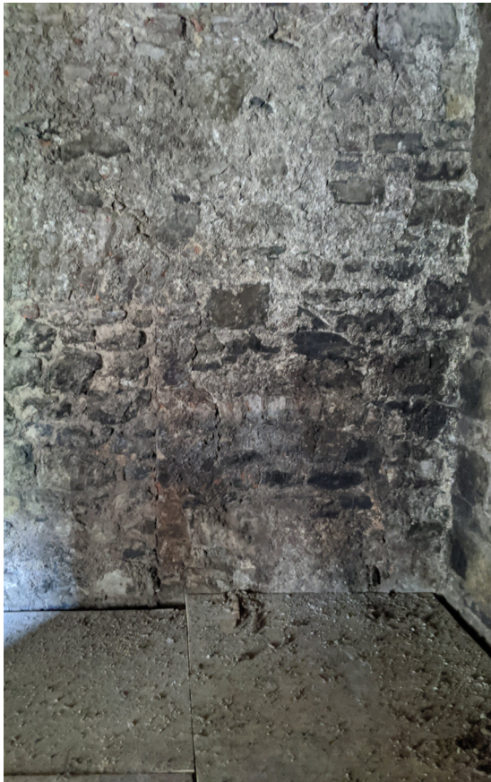
Figure 2.42 Northwest corner Breaks in bond of stonework suggest former openings (Refer Section C-C')
