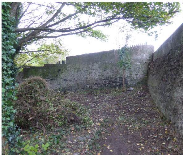
Figure 3.60 The wall has been built up in concrete blockwork at both boundaries
