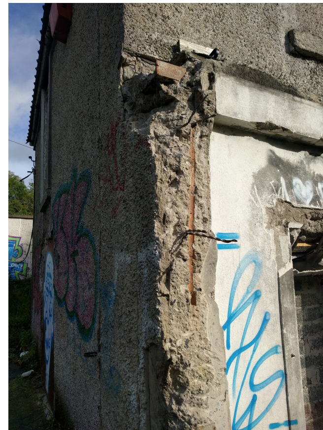
Figure 3.15 South Elevation 18th C wings Remaining reinforced concrete from the demolished 20th century single storey structure.
