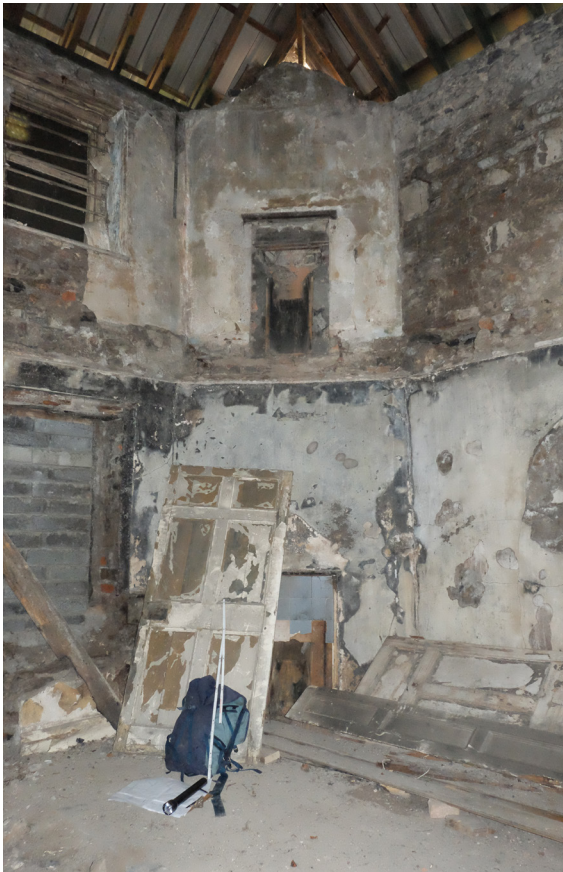
Figure 2.36 Northwest corner. Apex of chimney breast at former ceiling level. 19th century fireplace at upper level.
