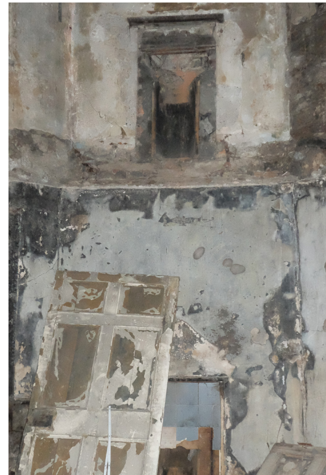
Figure 3.32 Room 18-04: upper floor cast-iron fireplace, tiled fireplace in poor condition below
