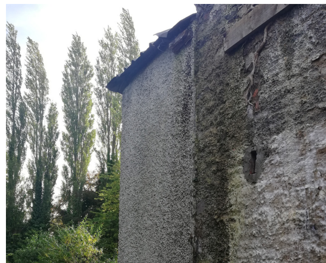
Figure 3.12 North Elevation Evidence of pockets in wall for structural timbers to demolished 20th century two storey structure.
