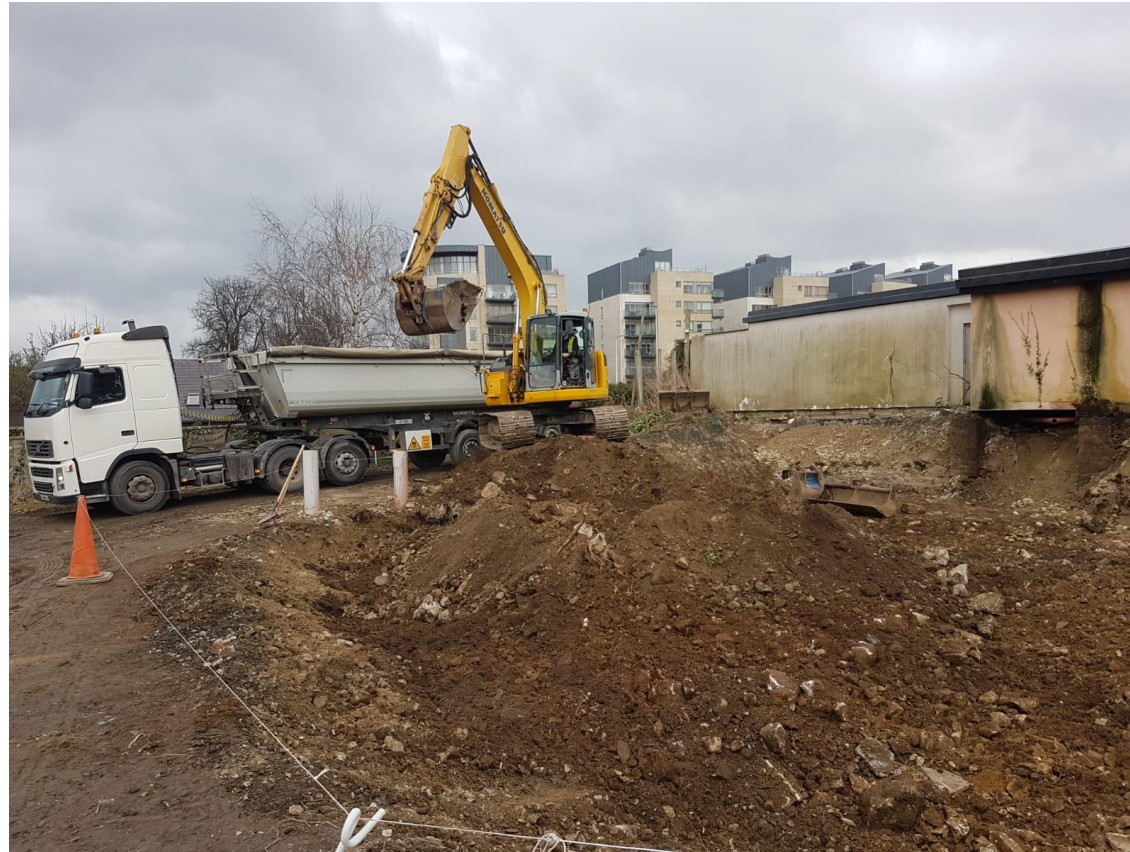
Excavating Japanese knotweed-contaminated soil from a development site
