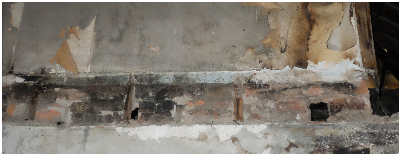
Figure 3.17 Evidence of rafters in brick & timber partition wall between Rooms 18-02 & 18-03
