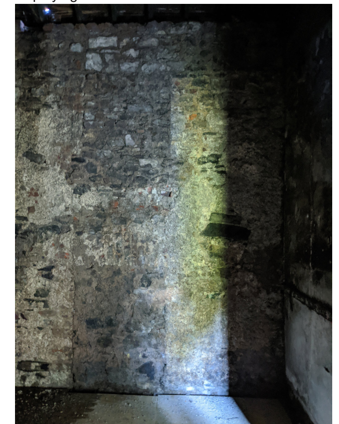
Figure 3.21 Random rubble walls to room 19-05 Evidence of openings in formerly external wall
