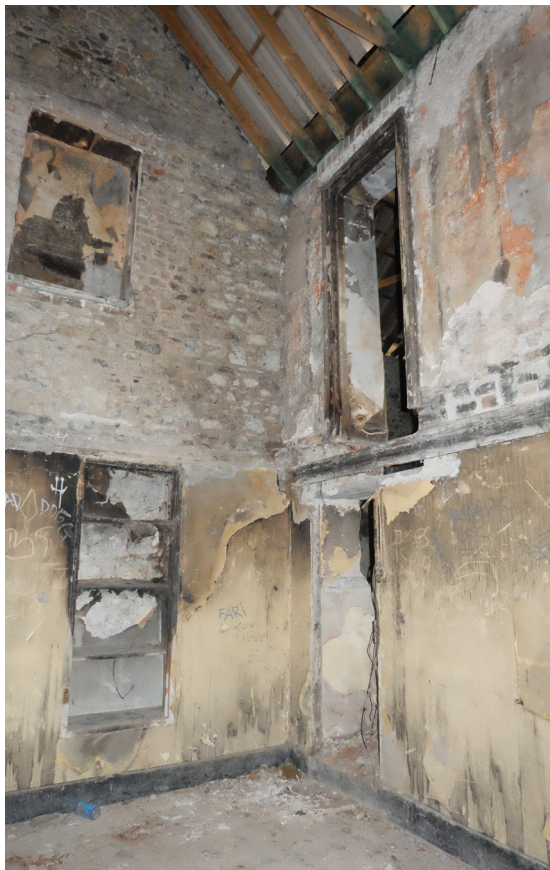
Figure 2.20 Northeast corner Doorway at upper level is at half landing level of the former stairs. Storage recess in north wall.
