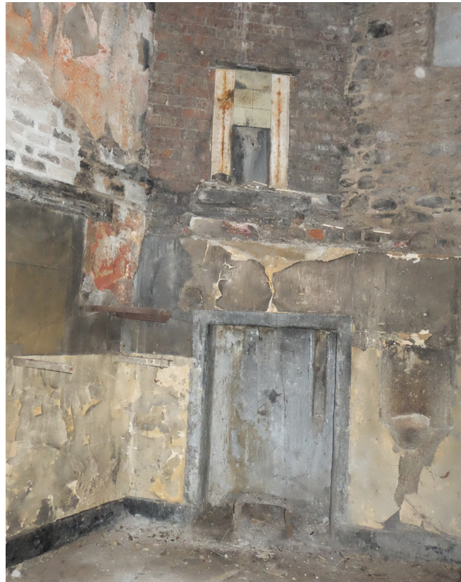
Figure 3.28 20th C tiled fire place at upper floor, limestone fireplace at lower floor in room 18-01.
