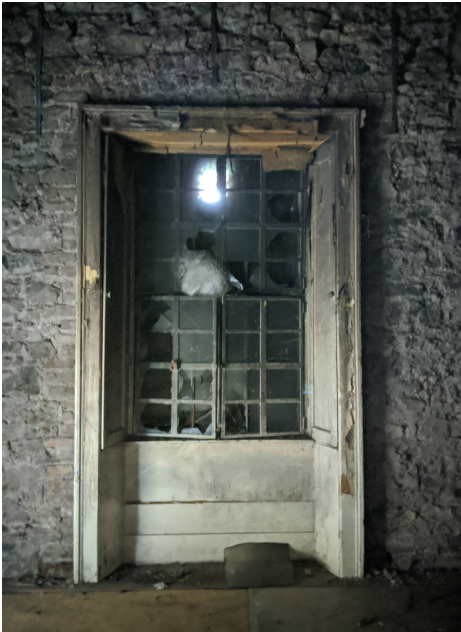
Figure 3.35 Sash window, timber shutters, and steel secondary glazing Room 19-05
