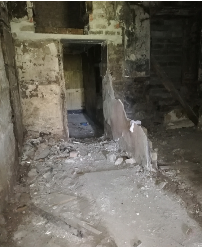
Figure 3.23 Edge of concrete slab at former stair / corridor space Room18-03
