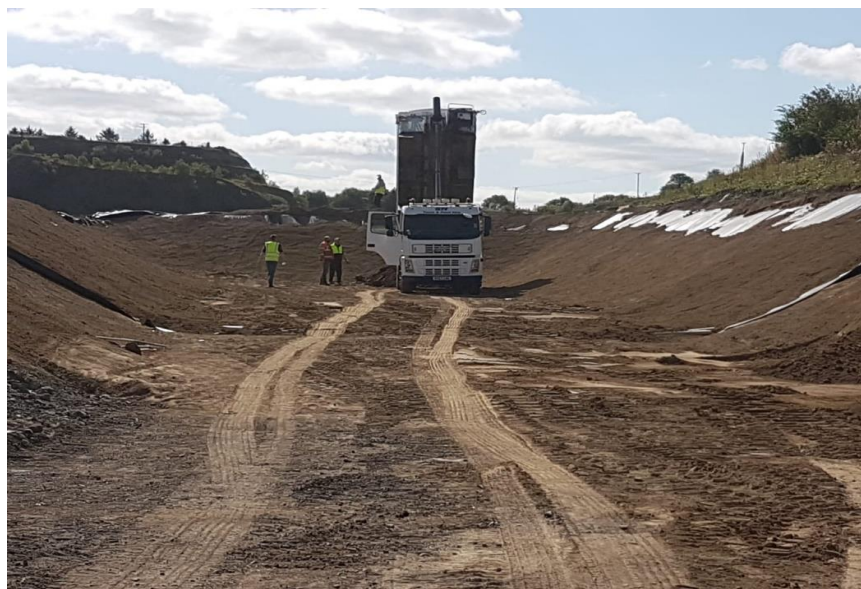
Depositing contaminated soil in deep burial site
