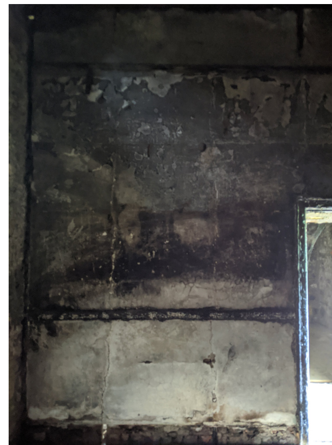
Figure 3.20 Brick noggin partition, Room 19-05 Sections of historic dado picture rail and architrave
