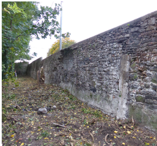
Figure 3.61 Note the rounded boulders of the rubble stone construction, and the hole repaired with concrete block.
