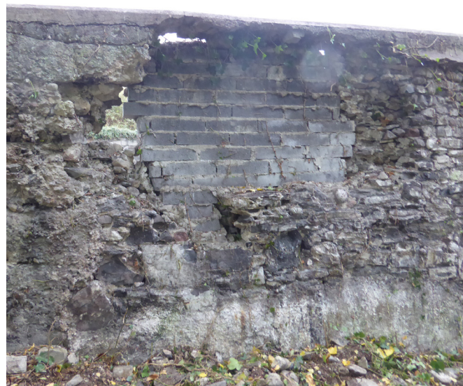
Figure 3.67 Collapsed wall at junction of rubble and mass concrete, repaired with blockwork
