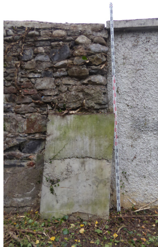
Figure 3.62 Buttress at junction of old and new walls
