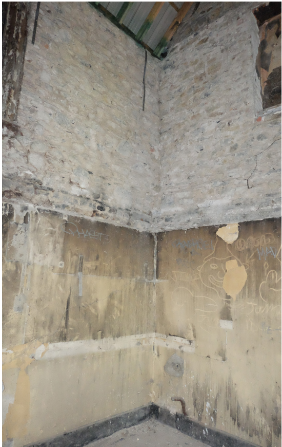
Figure 2.24 Northwest corner Plaster at ground floor is finished with a gloss paint suggesting use as a kitchen or dairy
