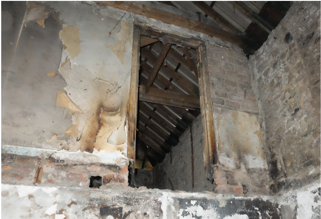
Figure 2.26 North wall: Brick & timber partition with room 18-03. Surviving architrave at upper floor.
