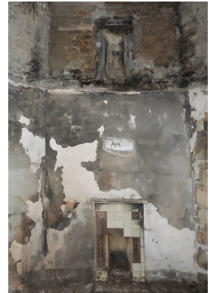
Figure 3.33 Room 18-02: upper floor fire place lost, lower floor in very poor condition.
