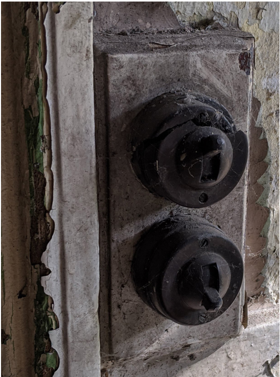
Figure 2.48 Room 19-06 Bakelite light switches
