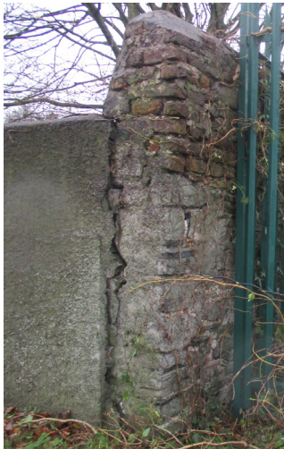
Figure 3.53 Open joint at corner
