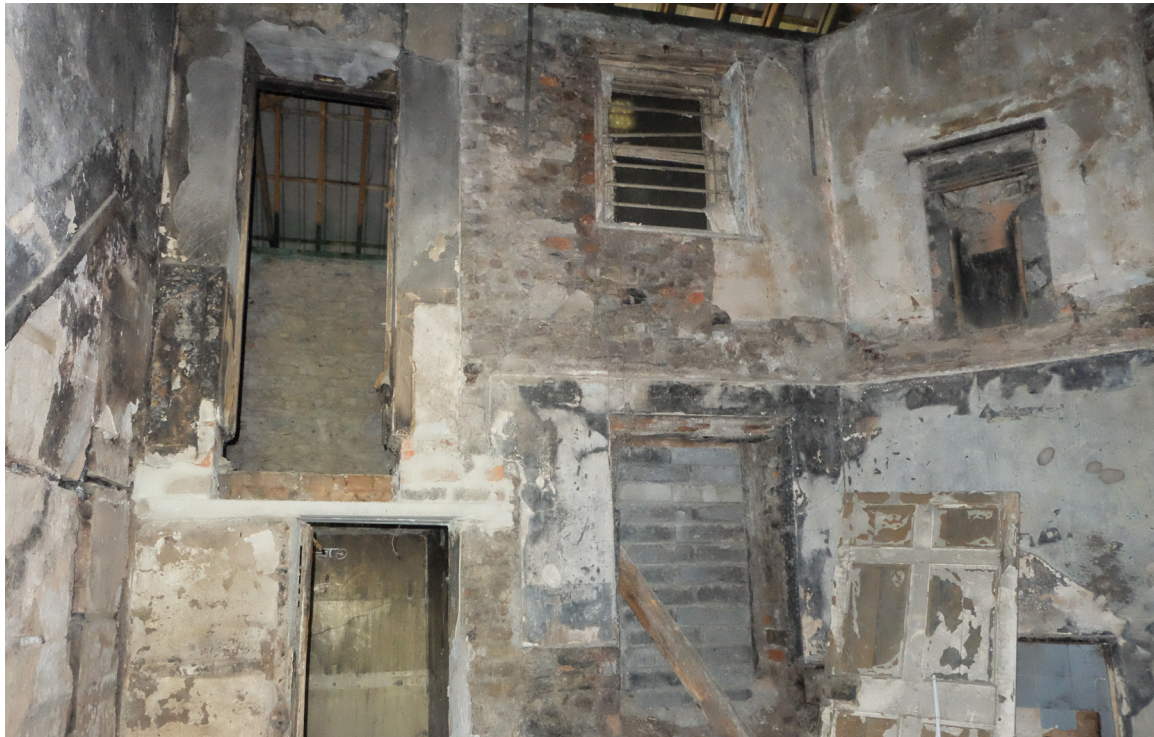
Figure 2.32 West wall See modern pre-cast lintel at door into Room 18-01 . 20th century window at upper level. Blocked window at ground level
