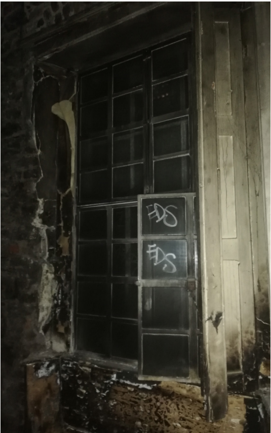
Figure 2.45 East wall Steel secondary glazing
