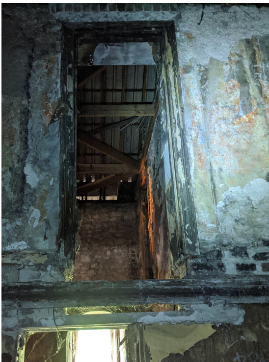
Figure 2.18 Modern precast lintel below timber that runs at former cornice level
