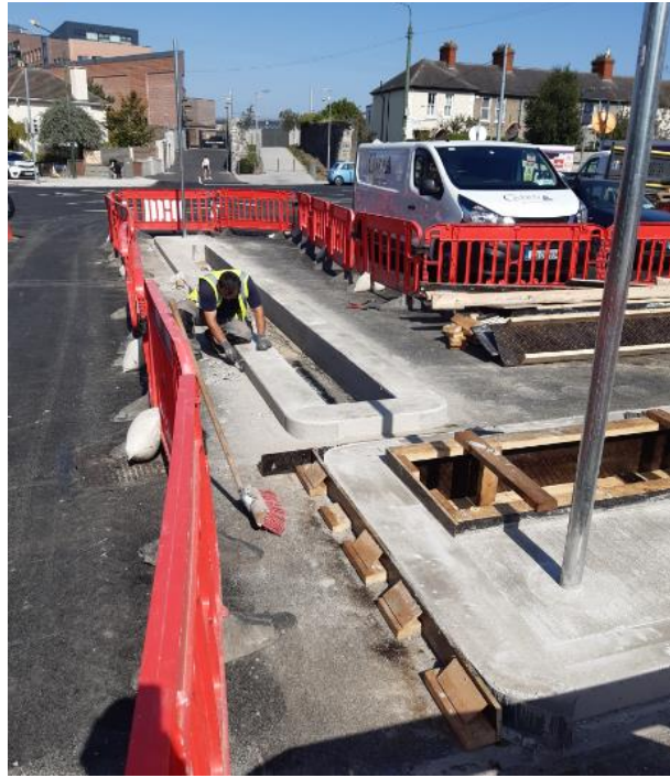
Construction underway on concrete buildouts with planting / landscaping at the filtered permeability location.
