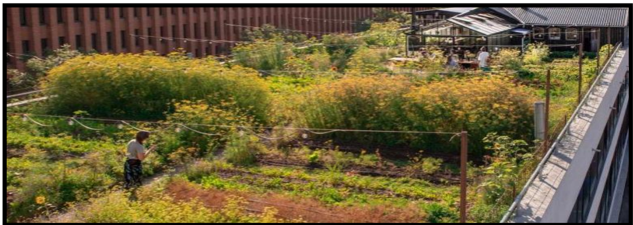
Green roof in Copenhagen
