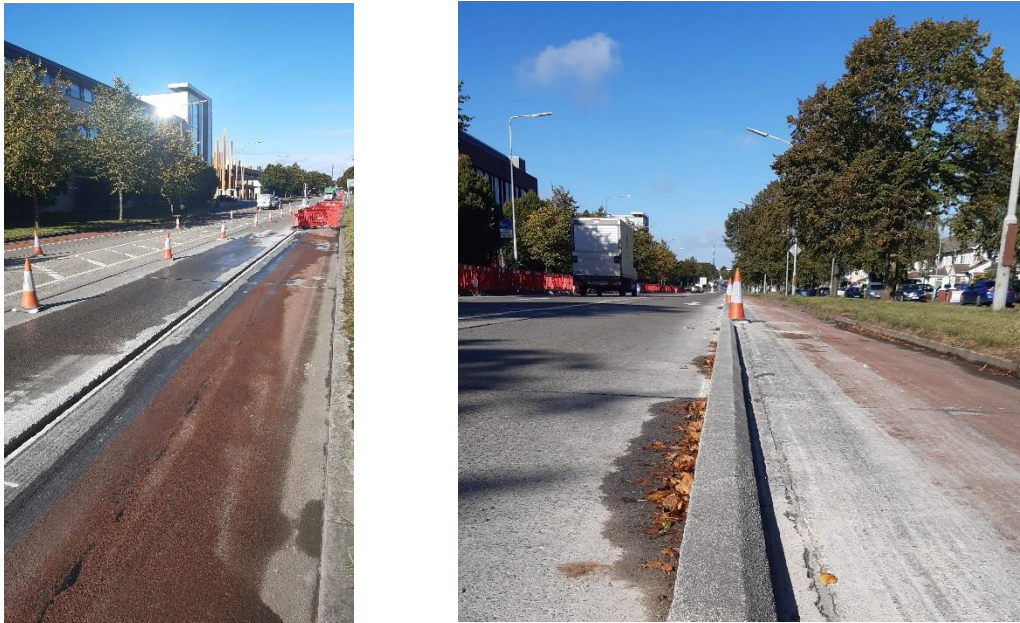
Works underway on Collins Avenue Cycle Route
