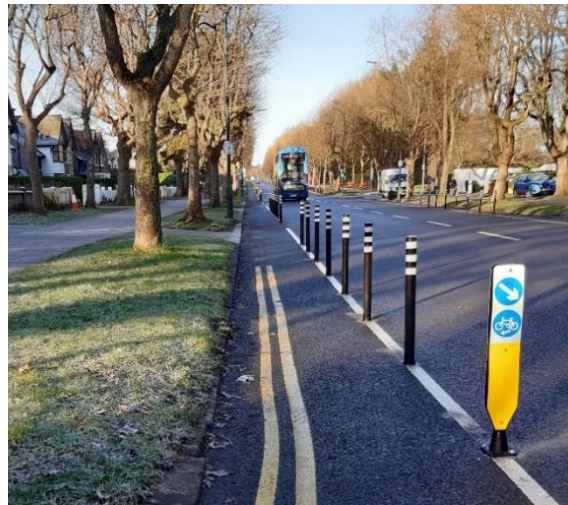
Road markings and protected cycle lanes between Walnut Rise and the Swords Road.
