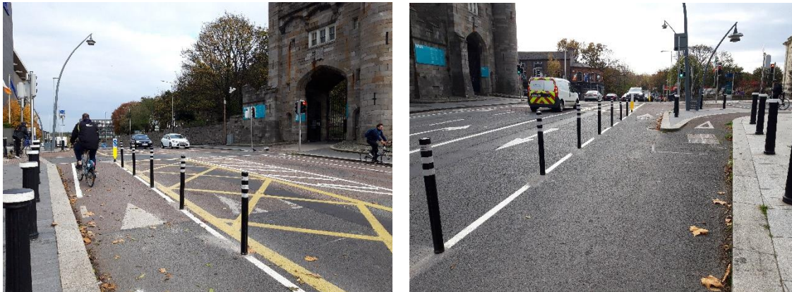
New protected cycle lane southbound passing entrance to Royal Hospital Kilmainham on South Circular Road
