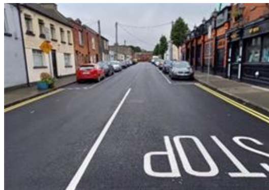
Completed resurfacing works
