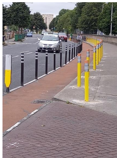
Protected cycle lane into a School Zone outside St Gabriel's National School Ballyfermot Dublin 10
