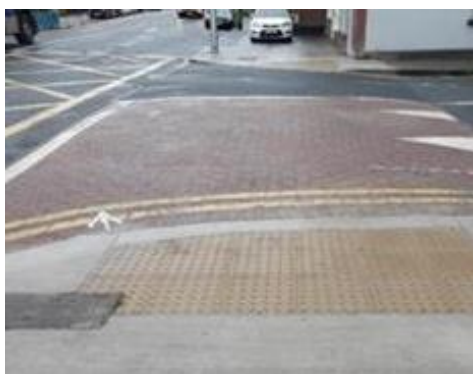
Tactile paving Monck Place / Phibsborough Road junction
