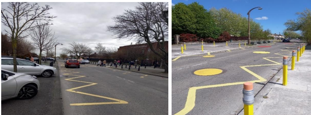
Armagh Road Crumlin before and after School Zone installation
