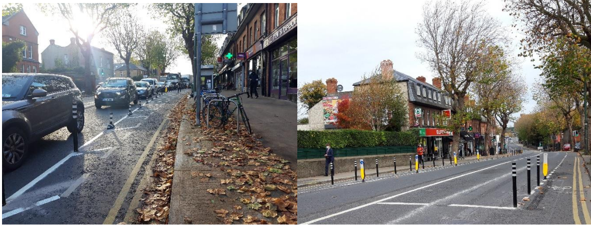
New protected cycle lane north and southbound outside shops on South Circular Road
