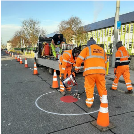
Improved Techniques in Colourful Circle Road Marking from painting direct to road surface to use of adhesive for made to measure circles
