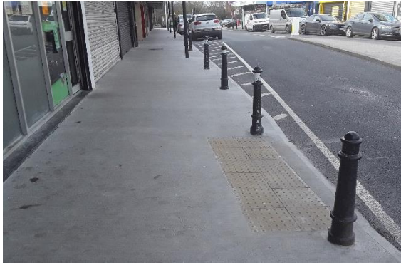
Footpath upgrade, Main Street, Finglas Village
