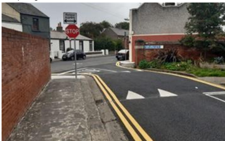
Entry treatment ramp on Great Western Square at the Great Western Square / Monck Place junction.
