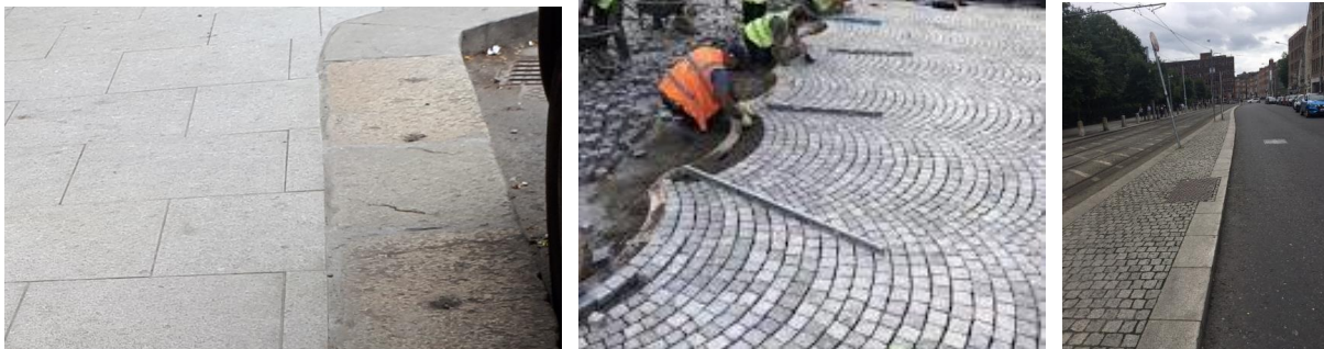
Granite slabs and kerbs, Bogen pattern paving and granite details.
