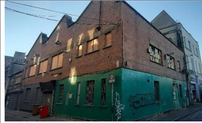
Fig. 3: Nos. 4-8 Henry Place - view from northeast
