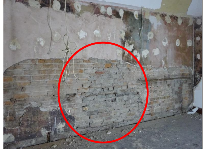
Fig. 8: Second Floor rear room of No. 10 with repaired brick work in the party wall to No. 11 as evidence of a 'creep hole' made during 1916
