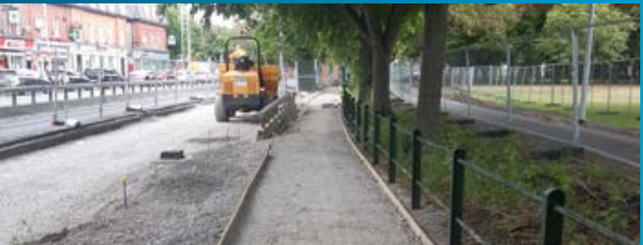
Fairview Cycle Track under construction.
