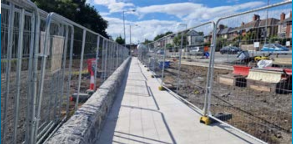
Clontarf Road Footway & Stone Wall alongside Fairview Park.
