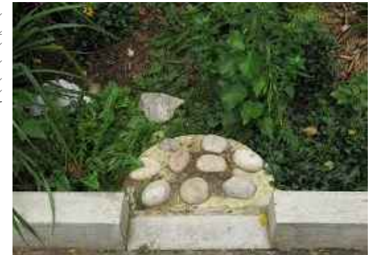
(Above) Example of a Kerb-cut Inlet detail, with cobbles embedded in concrete, to slow the speed of surface water draining into the rain garden (coming from a transverse fall across the carriageway), to prevent soil erosion and scouring.
