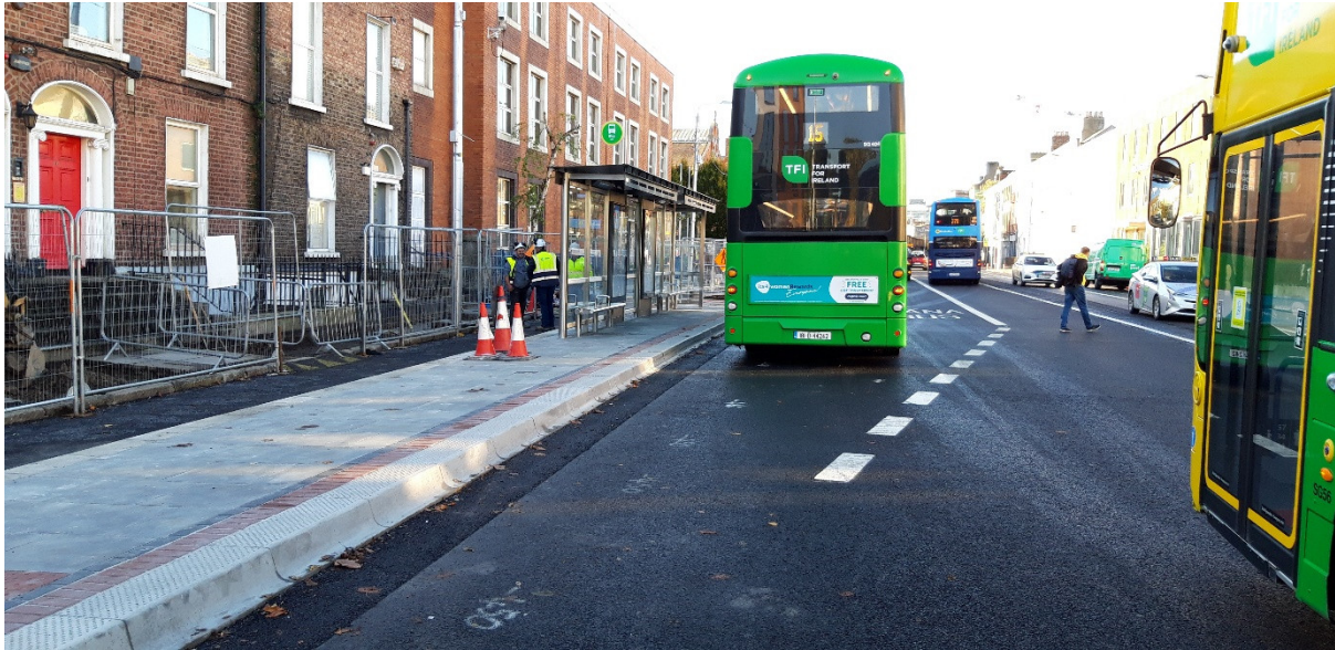
Figure 7.1: Bus Stop 619 Amiens Street near Portland Row (Photo 26/10/2022)
