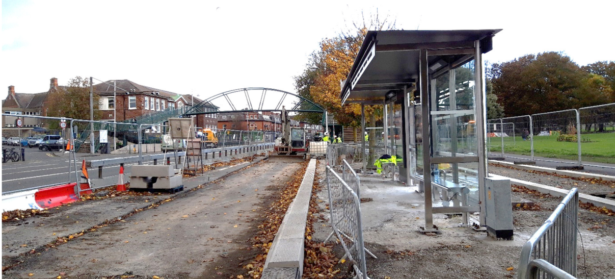
Figure 7.2: Bus Stop 614 Footbridge at Fairview (Photo 26/10/2022)
