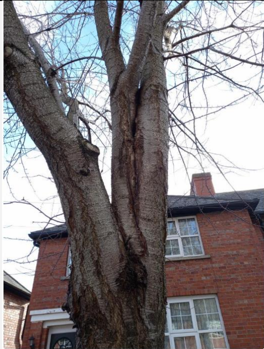
Prunus avium (Wild Cherry tree) at 64 Iveagh Gardens. Compression fork with included bark. Two cracks in limbs. Large limb failure to be expected at fork.
