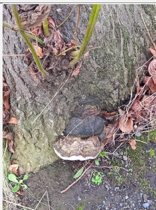
Ganoderma: Decay Fungi growing at the base of Lime tree at 103 Iveagh Gardens.
