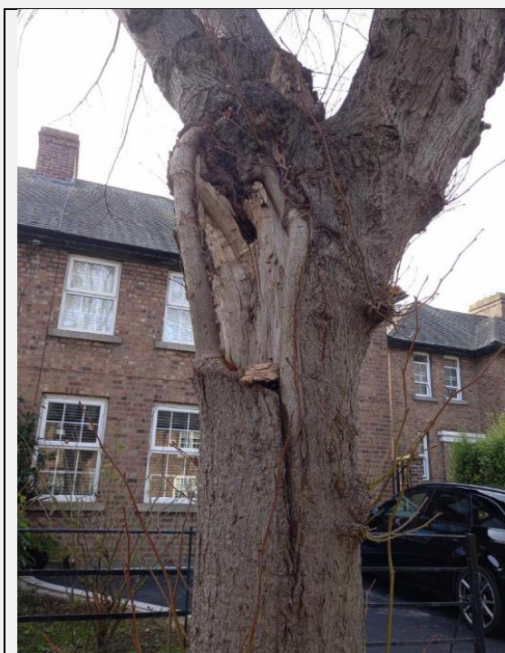
Tilia x europaea (Common Lime Tree) with large cavity due to branch failure at 103 Iveagh Gardens.
