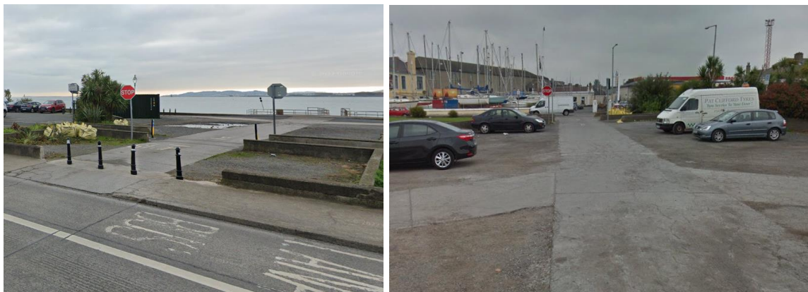
Figure 2 Boat Access to Slipway from Clontarf Road (South),
