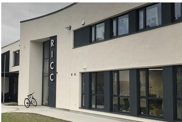
Refurbishment of Ringsend and Irishtown Community Centre.
