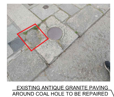
EXISTING ANTIQUE GRANITE PAVING AROUND COAL HOLE TO BE REPAIRED
