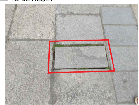
EXISTING LOOSE FLAGSTONE TO BE RESET
