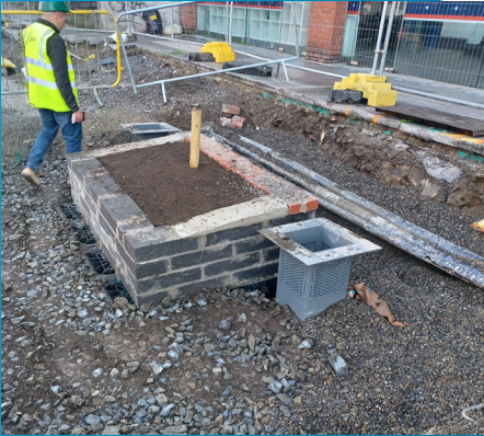
Bespoke designed tree pits are being installed to support new trees on the scheme
