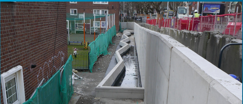
New retaining wall constructed at James Larkin House with areas for future planting
