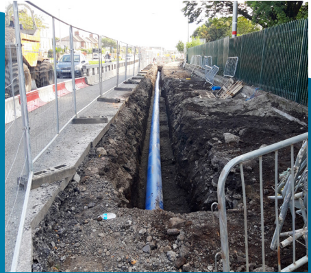
Approximately 6km of 100 year old watermain are being replaced throughout the route
