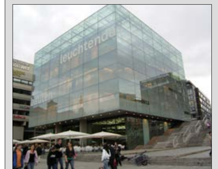
Figure B4.4. Belmayne Square (and Belcamp Square) will cater for a range of outdoor activities (top, middle). A civic/cultural building will also be located within Belmayne Square at a location where it will be highly visible and provide a degree of shelter from westerly winds.
