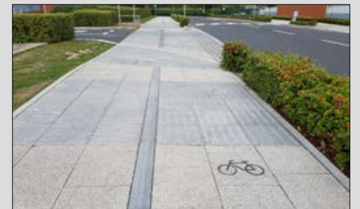
Raised entries and/or continuous material treatments at side street junctions will slow turning traffic vehicles and prioritise movement for cyclists and pedestrians.
