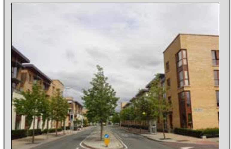
Tree planted median creates an attractive boulevard like environment, which promotes greater enclosure of the street (traffic calming) and provides an area of pedestrian refuge.
