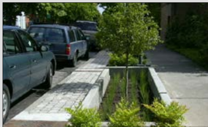
Example of Sustainable Urban Drainage swale which also provides an attractive landscape feature.
