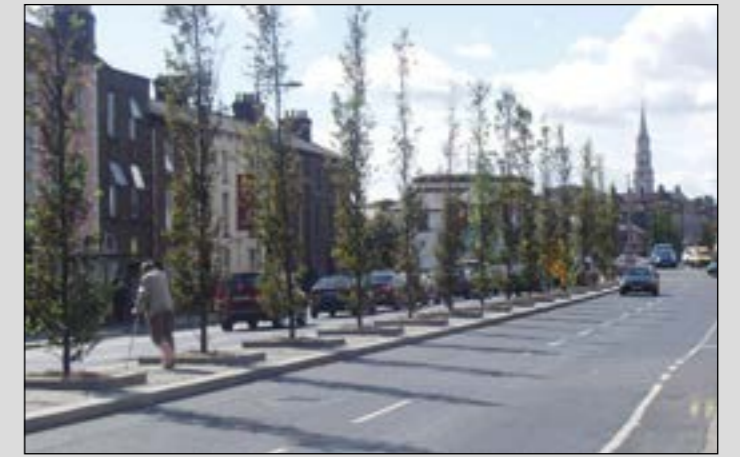
A tree planted median along the Main Street will create an attractive boulevard like environment, promote a greater sense of enclosure (traffic calming) and provide an area of pedestrian refuge.
