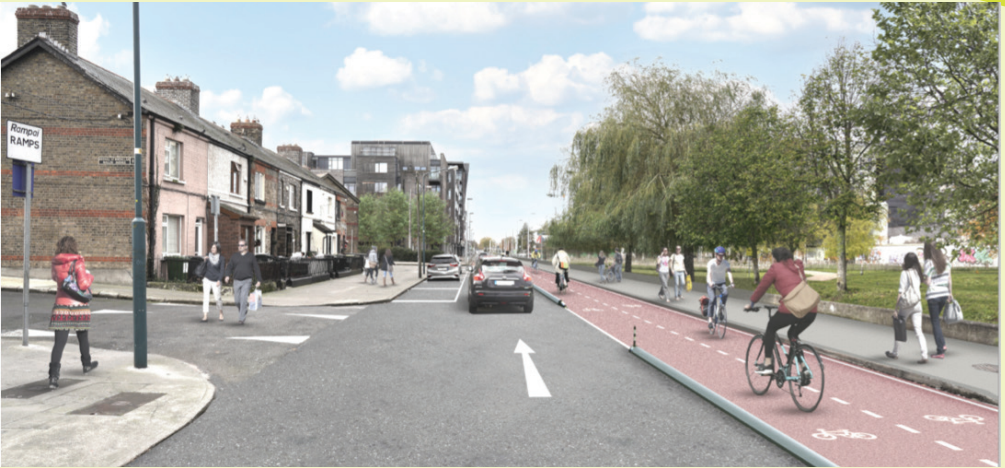
Two way protected cycle track on the North side of James Walk
