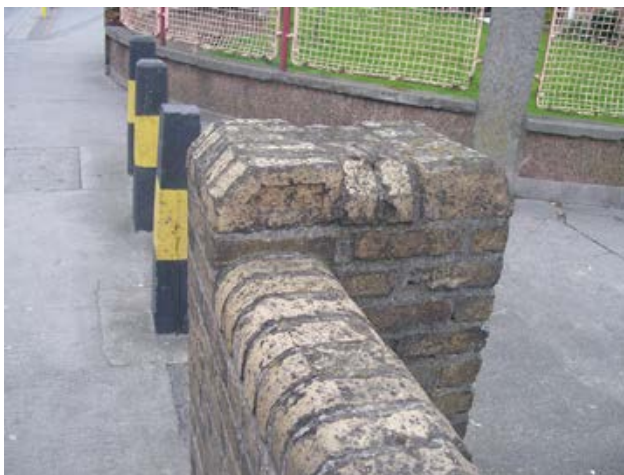
DBC Brick Wall, Crumlin Road (Courtesy of John Buckley)
