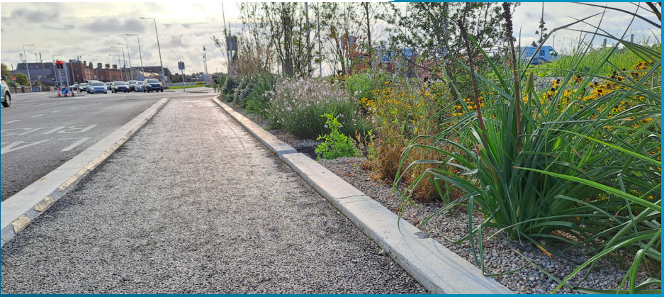
Paving and landscaping along the route continues
