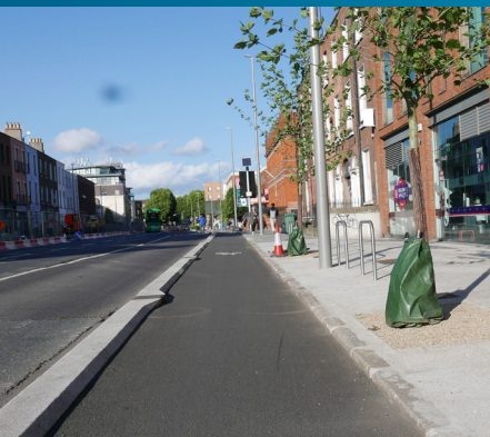
New Paving, Planting and cycletrack in public use
