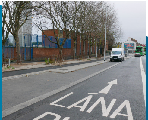
Public Parking opened and Sustainable Urban Drainage Bio Retention areas in operation at North Strand Fire Station
