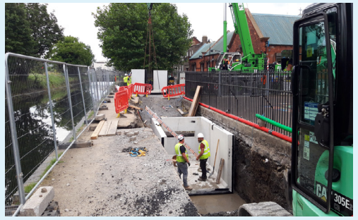
Bá ailt cábla ardvoltais leictreachais a shuiteáil gar do Mheal Charleville
