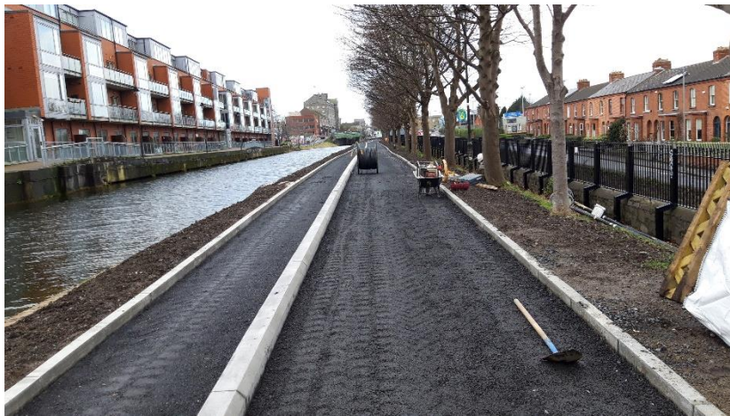
Kerbing installed on north side towpath between Cross Guns Bridge and lock 4
