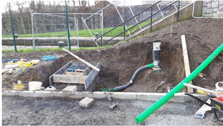
Installing CCTV ducting & chambers at Lock 4
