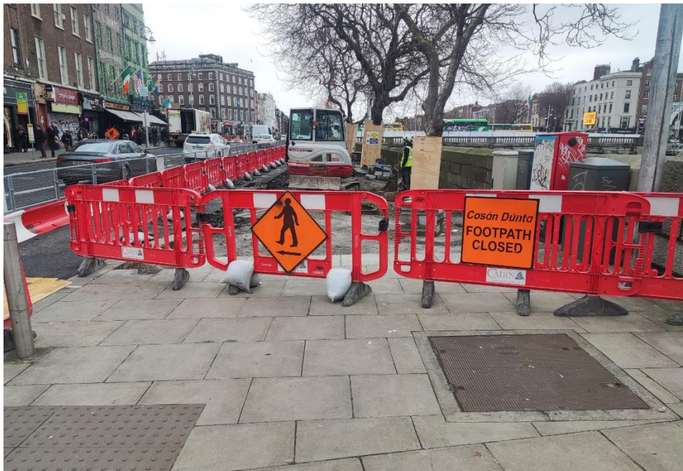
Works commencing on Burgh Quay
