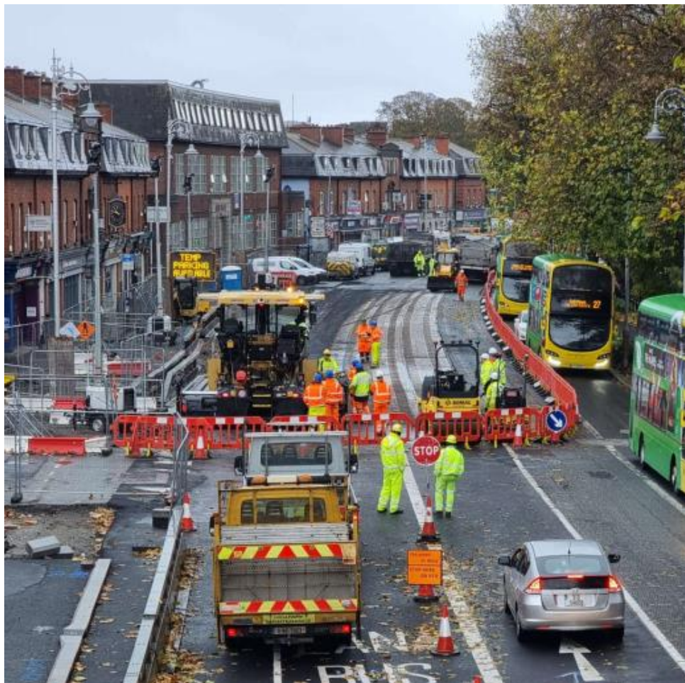
C2CC – Road Construction works through Fairview Village (weekend works)
