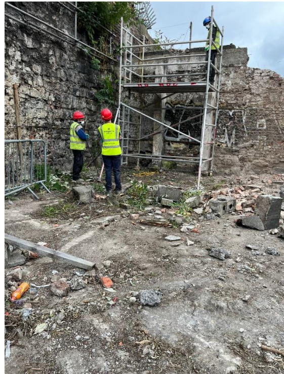
Plate 45 The removal of brick by hand at Wall 2 abutting the City Wall
