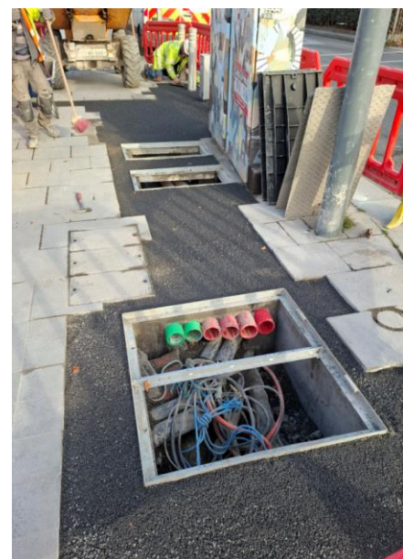
New chambers and ducting at the corner of Whitworth Road & Drumcondra Road Lower
