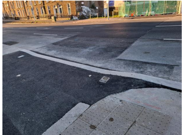
Temporary reinstatement of footpath and carriageway at Clarke's Bridge
