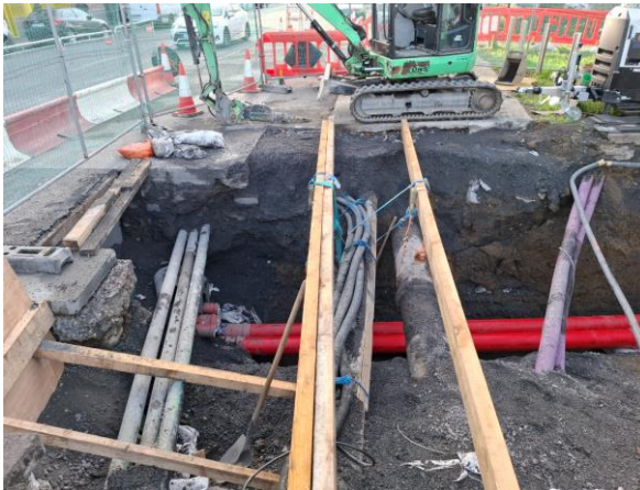
High voltage electricity ducting being laid underneath existing utilities at Clarke's Bridge
