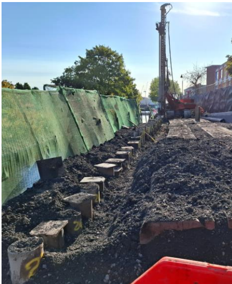
Piles being driven between Clarke's Bridge & Charleville Mall
