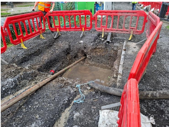
Launch and reception pits for horizontal directional drilling underneath Dorset Street Lower
