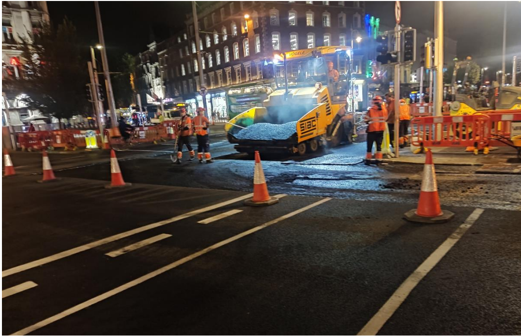
Night time resurfacing works at O'Connell Bridge junction.
