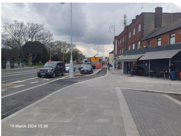
C2CC – Footway, paving and raised table pedestrian crossing at Merville Avenue and Amiens Street Outbound (cycle-track opened 19 th July 24)
