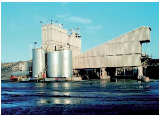
Figure 3.15. Energy efficient asphalt plant incorporating insulated bitumen tanks and aggregate bins (Roadstone Provinces Ltd, Bunratty, Co. Clare).
