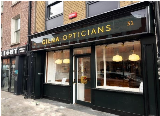
Recently completed shopfront renewal at 31 Thomas Street
