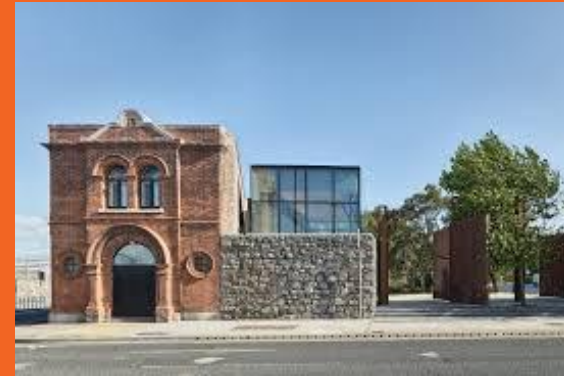
Dublin Port Substation
