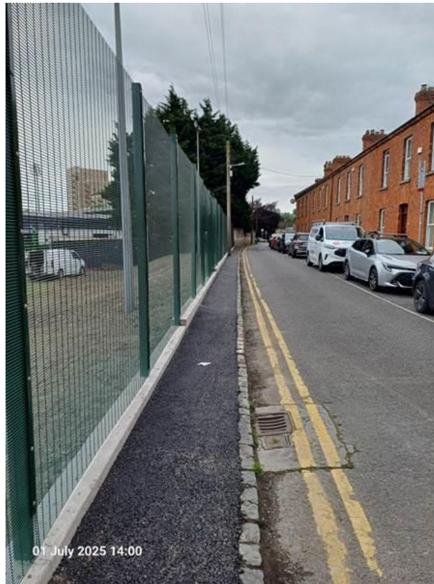
Figure 6 -New fence on Eglinton Terrace
