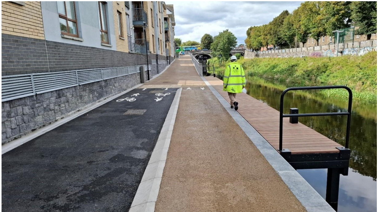
Figure 2 – upgraded jetty, and new facility near Binns bridge
