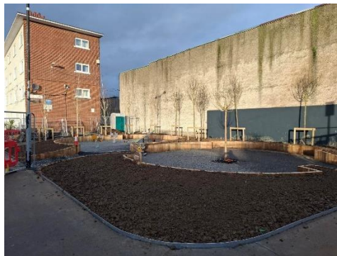
Playground upgrade works progress (1 st November and 27 th November)
