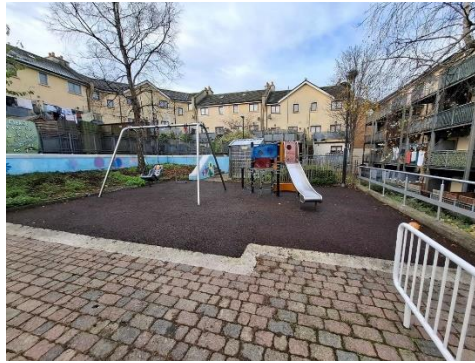
Playground upgrade works (before and after).
