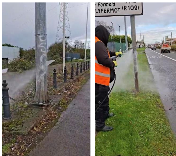
Naas Road– Graffiti removal and general clean up
