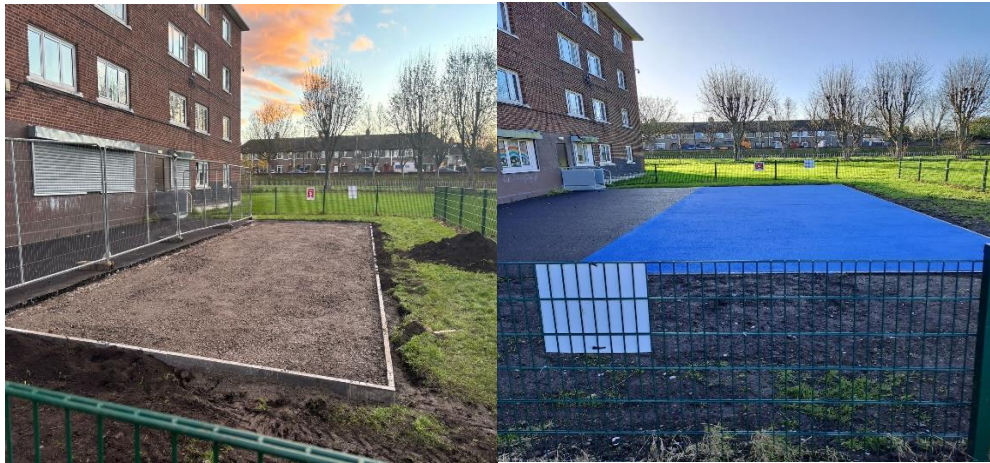
Dolphin House New Soft play area installed at Creche
