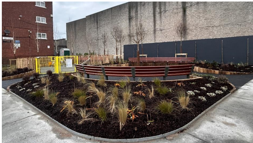
Work was completed at the end of December on the development of a new pocket park at Vicar Street
