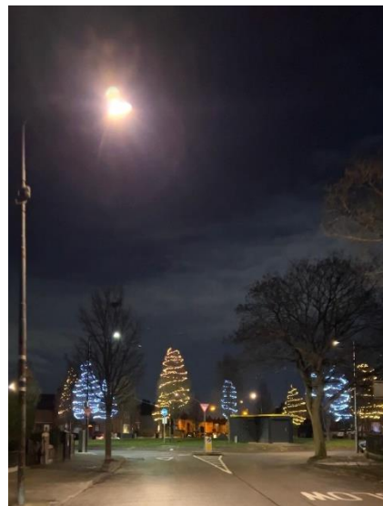
Tree Lighting installations at Mourne Rd.
