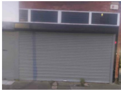
Shutters on Emmet Rd had Graffiti painted out.
