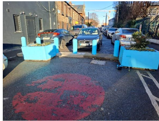
Basin View Re-instatement The Hoarding was removed in December and Road Maintenance re-instated the planter and bollard. The area has been power washed and all the street furniture re-painted as an interim measure
