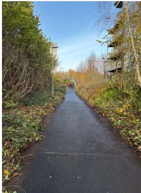
Removal of overgrown vegetation on path connecting Castleview Apartments to Lansdowne Gate, Bluebell
